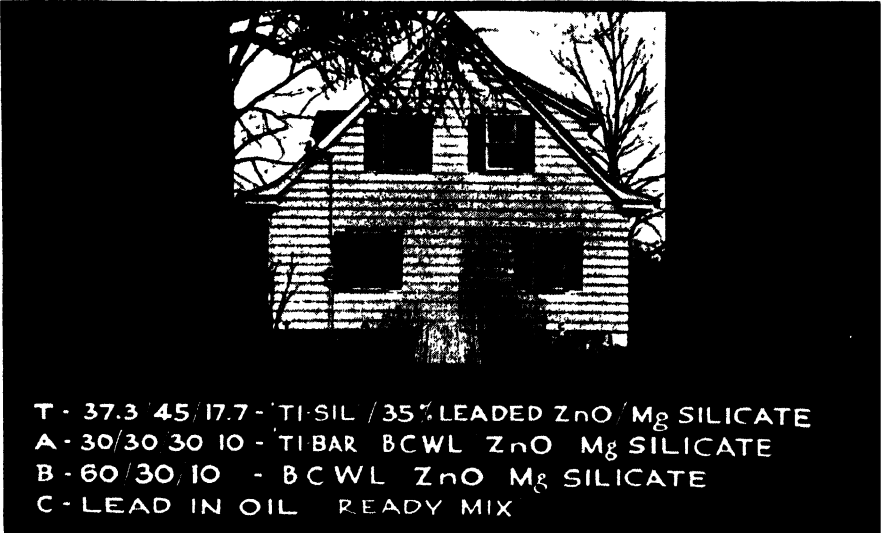
FIGURE 20. Delaware west vertical—4½ years—white repaint.
