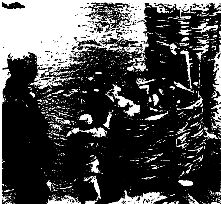
CHINESE WEIGHTED WOVEN PIERS WITH STONES TO BUILD A BRIDGE.
