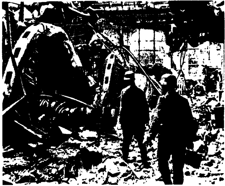
GERMANS BATTLED INTO A POWER PLANT, REDS DUG IN AGAIN BEHIND IT
