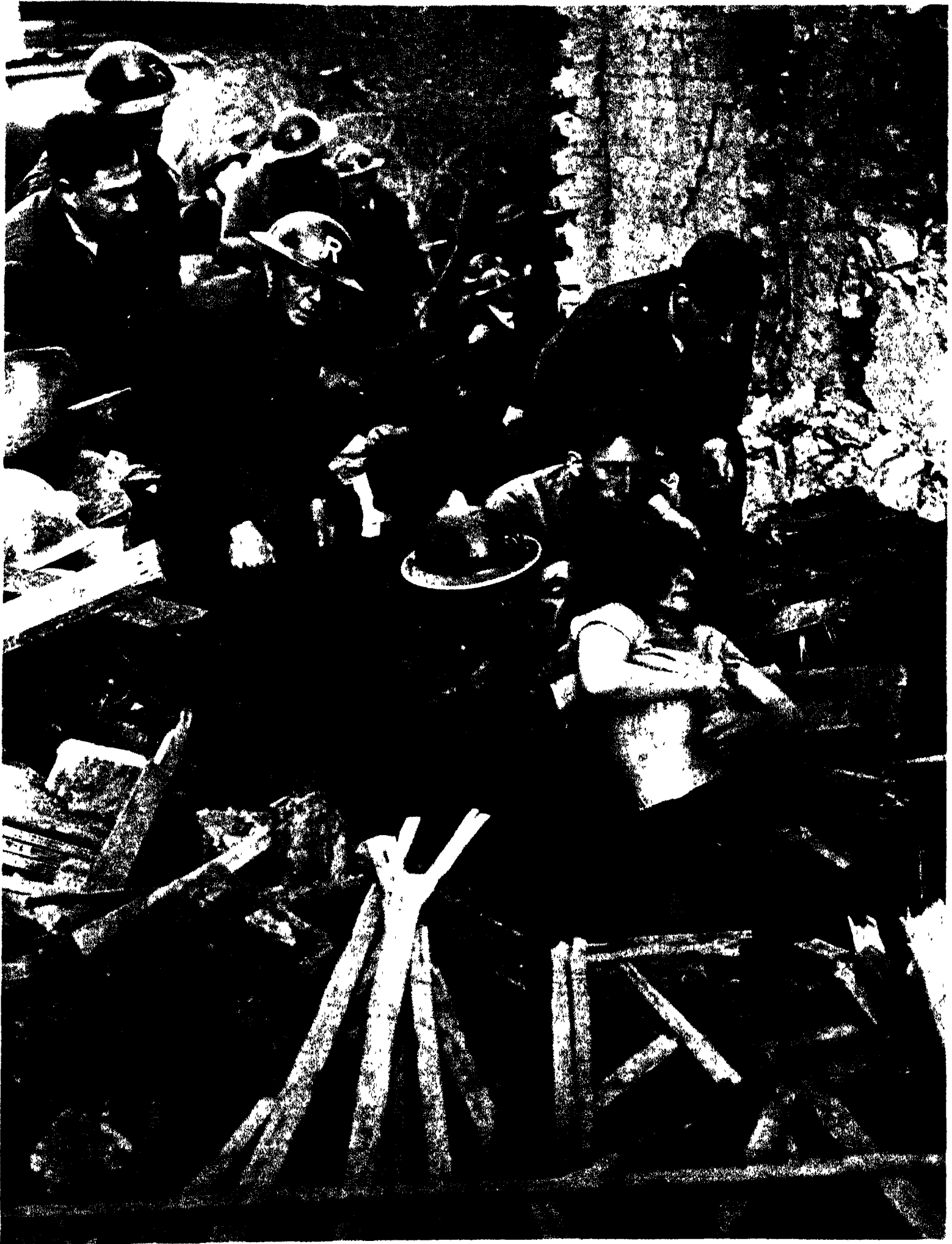
RESCUE OF A WOMAN from the basement of her bomb-collapsed house came after 18 hours of digging. This was one of 50,000 bomb "incidents" during the blitz which kept Londoners constantly probing through the
