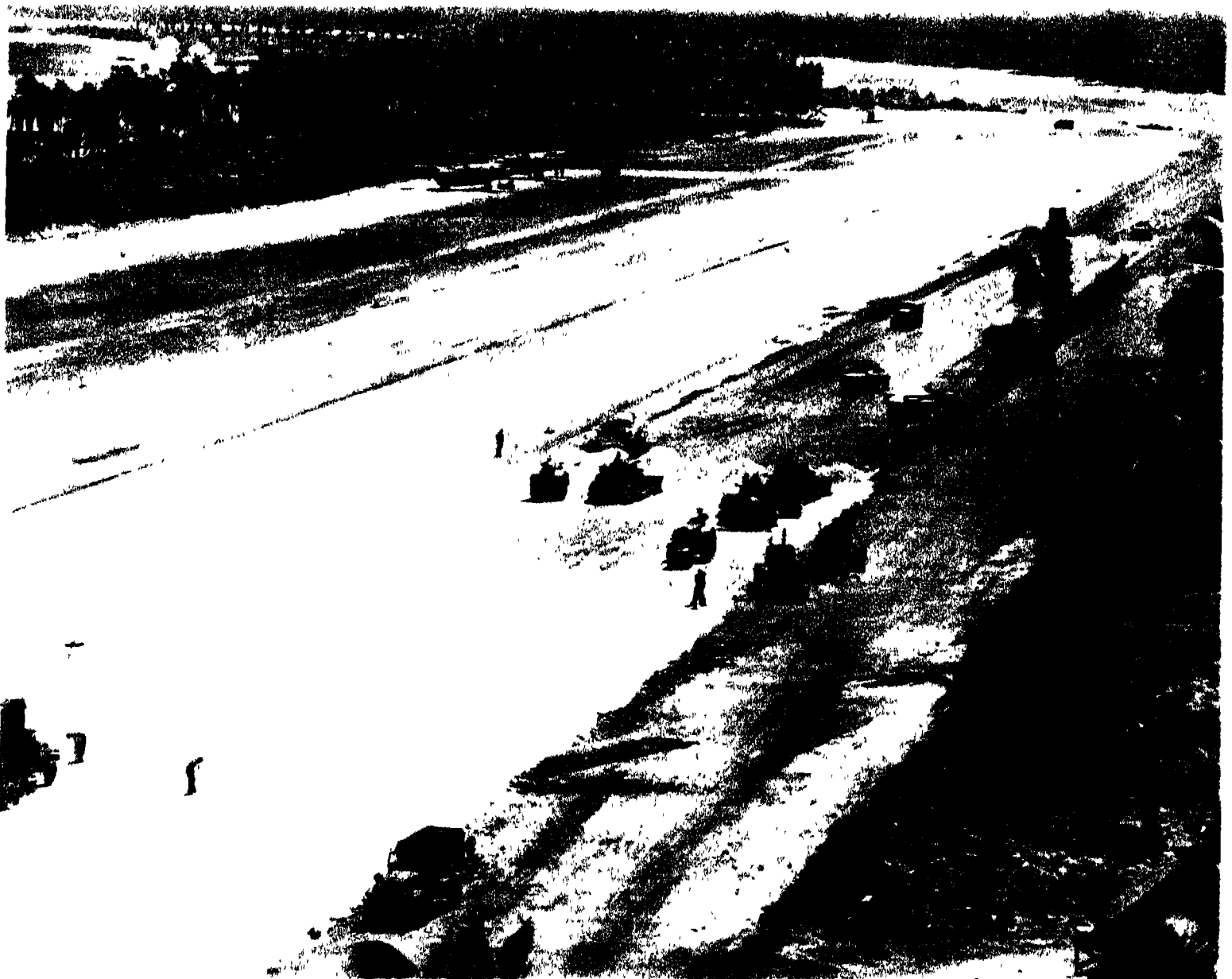
A FEW DAYS AFTER ENIWETOK FELL SEABEES HAD CLEARED AN AIRSTRIP FOR U.S. BOMBERS, SOON WERE WIDENING IT (ABOVE) FOR MORE TO COME
