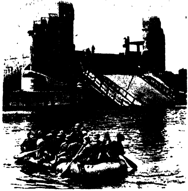
DENIED A BRIDGE at the frontier by Dutch dynamite, Nazi engineers crossed the river in rubber boats. Paratroops seized intact the bridges leading to Rotterdam, held them open for the German ground forces.
