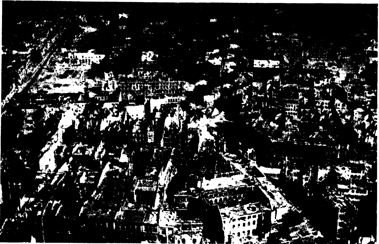
DURING 12 DAYS OF SAVAGE STREET FIGHTING IN BERLIN, RED ARTILLERY COMPLETED THE DESOLATION LEFT BY FOUR YEARS OF ALLIED BOMBING
