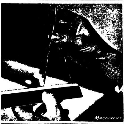
Fig. 8. Setting Compass to Given Radius
