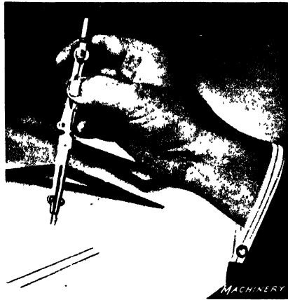
Fig. 7. Position of Hand for opening Compass readily when it is picked up from Drawing-board
