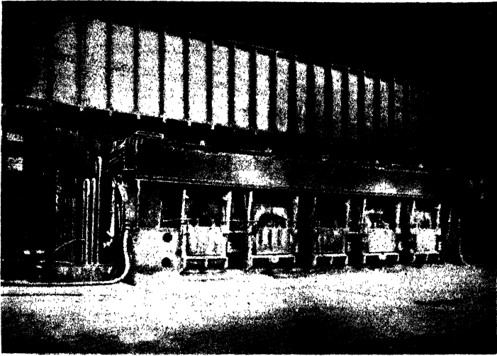
FIG. 18.—A 300-ton Tilting Furnace. Charging side showing Water-Cooled Doors.
