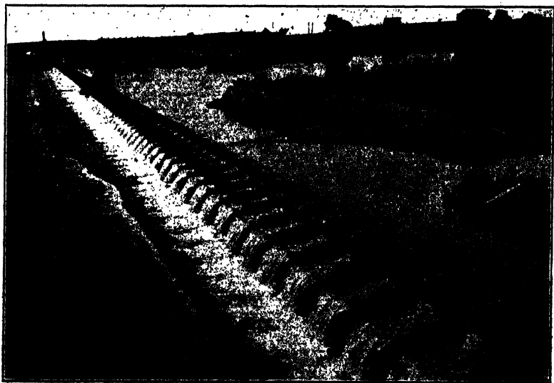
FIG. B.—Collapsible diversion weir of Prewitt Reservoir Project, Colo.
