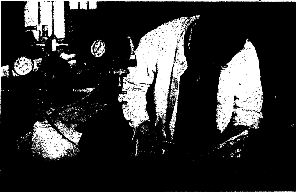
FIG. 46. OXY-ACETYLENE OUTFIT FOR LEAD BURNING IN USE ON SHEET LEAD
