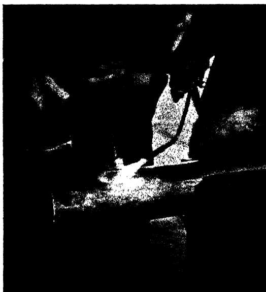
FIG. 65. FORMING A SOCKET FOR A BRANCH JOINT
