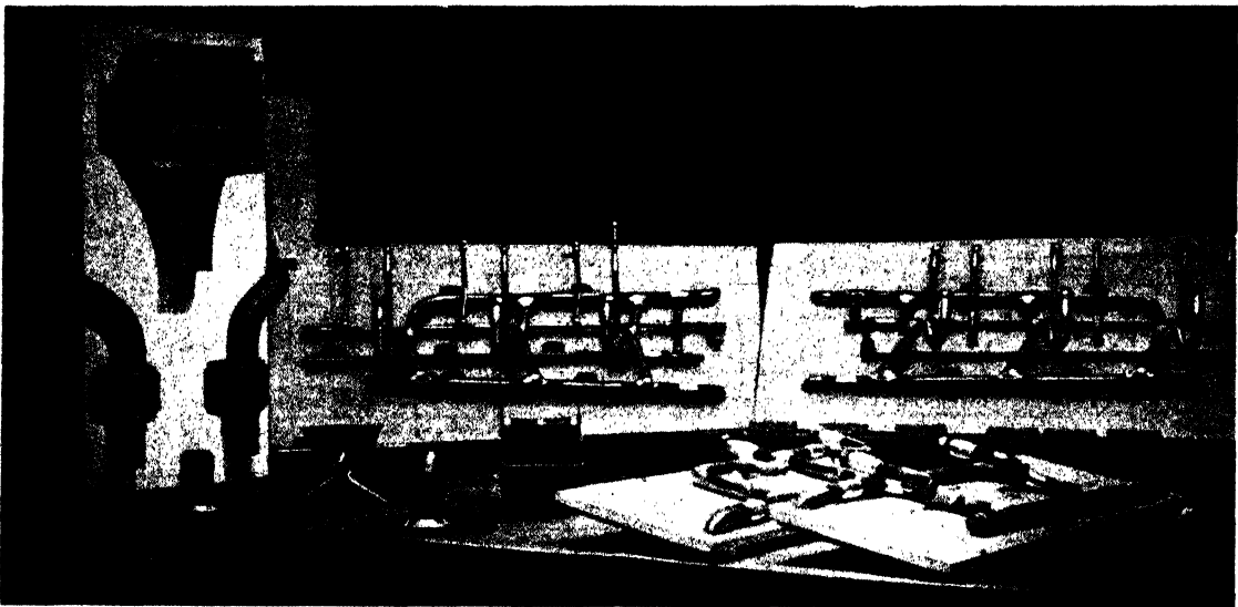
FIG. 179. WASTE, VENTILATION, AND COLD WATER SERVICE PIPES MADE UP READY FOR FIXING
