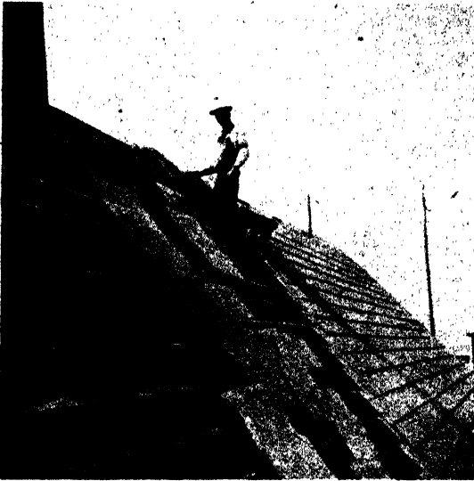
FIG. 10. BATTENED AND FELTED ROOF
