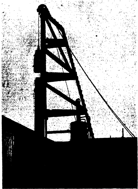
FIG. 140. LARGE PILE DRIVER
