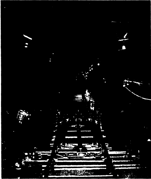
FIG. 90.—California Switch on Montebello water tunnel, Baltimore. The outside tracks are used for passing cars when mucking, but all heavy and wide equipment is hauled over the center track. Note the spring switches.
