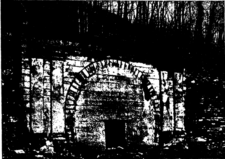
FIG. 4.—America's first railroad tunnel, Staples Bend, Allegheny Portage Railroad. Used for portaging canal boats over the Allegheny Mountains. Built 1831. ( Pennsylvania Railroad Photograph. )
