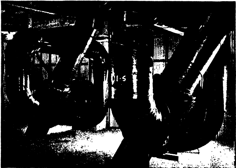
FIG. 143.—Two ventilating fans serving the north and south headings at Shaft 6, Delaware Aqueduct. The fans are nonreversible; direction of air flow depends upon position of the four-way valves. (Courtesy of Ingersoll-Rand Co.)
