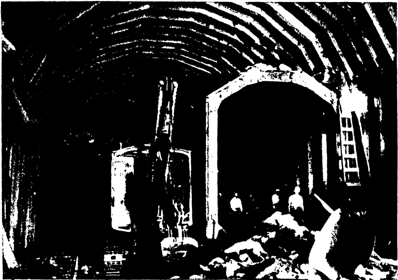
FIG. 279.—Double-tracking an old tunnel under traffic, Chesapeake & Ohio Railway. The traveling shield extended into the old single-track tunnel, protecting trains from the enlarging operations. (Courtesy of E. G. Rice, Chesapeake & Ohio Railway.)
