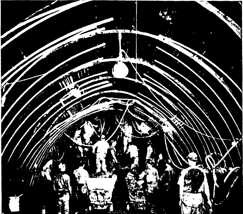
FIG. 202.—Ribs and plates in a Chicago sewer tunnel. As this was fairly good ground, plates were placed longitudinally to allow wider spacing of ribs. Reinforcing bars were set in the invert concrete which was carried to the face of the bench. (Courtesy of Commercial Shearing & Stamping Co.)
