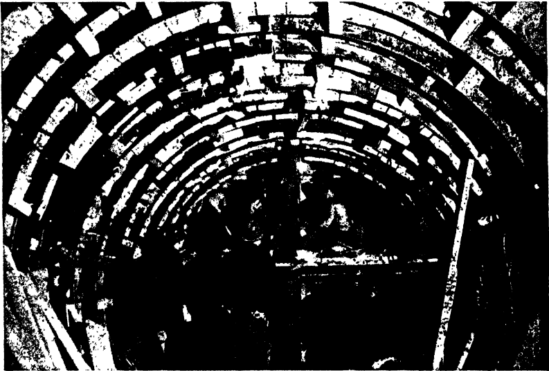
FIG. 323.—Forepoling dry running ground, Colorado River Aqueduct tunnels. Miners' scaffold is supported on pipes chained to ribs. ( Metropolitan Water District Photograph. )
