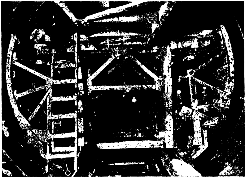
FIG. 332.—Steel wall forms, New York subways.
