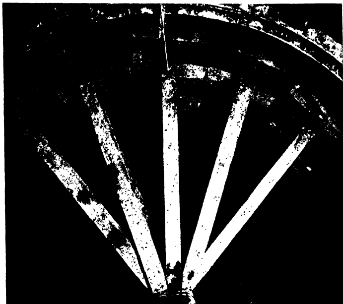
FIG. 184.—Needle-beam tunneling through Detroit soft blue clay. The advance end of the steel forms can be seen at the top.
