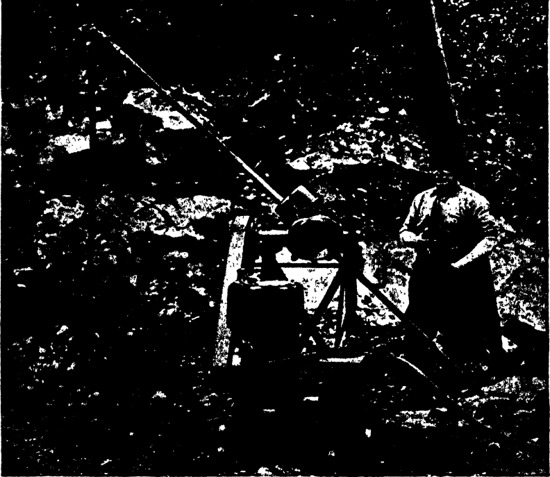
FIG. 15.—Diamond core drill making an inclined exploratory hole. (Courtesy Sullivan Machinery Co.)
