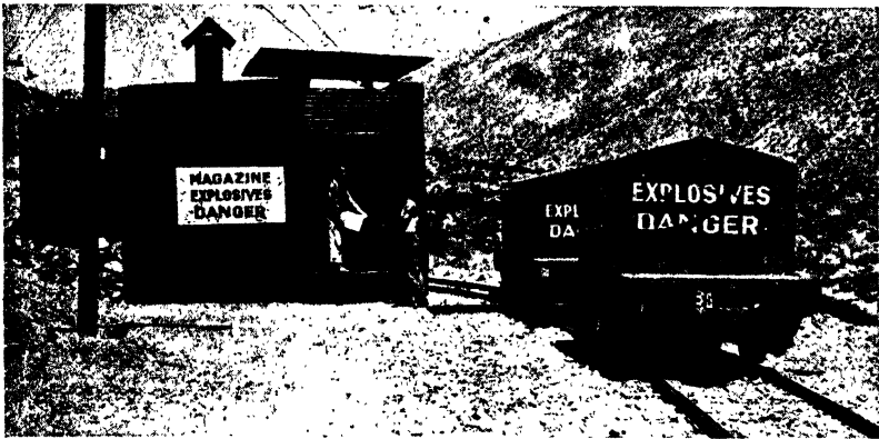
FIG. 302.—Magazine and explosives car used on Colorado River Aqueduct tunnels. ( Metropolitan Water District Photograph. )
