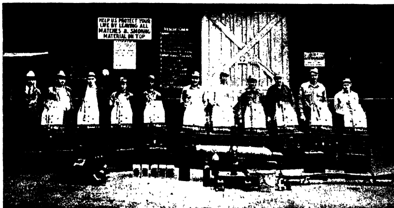
FIG. 54.—Rescue squad with special gas equipment, Hetch Hetchy Tunnel, San Francisco.
