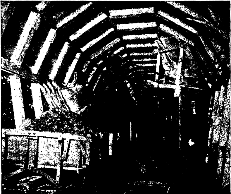
FIG. 319.—Five-piece arch sets with tight lagging. Note the inclined posts to resist possible horizontal pressures.
