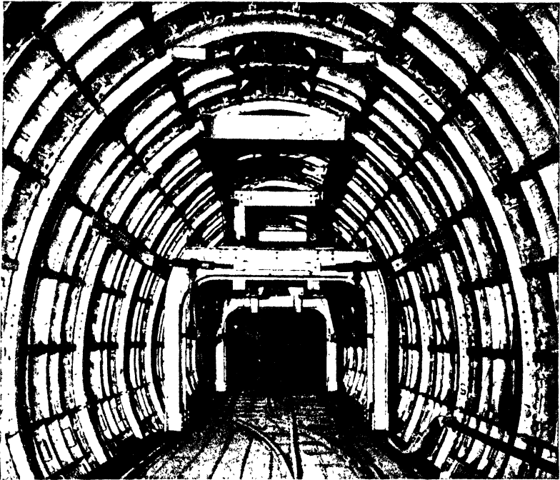
FIG. 329.—Telescoping steel forms, Chicago sewer tunnels. Usually the forms were handled on the traveler shown here, but in bad ground they could be dismantled and used as a rib-and-plate form around a needle beam. (Courtesy of Blaw-Knox Co.)
