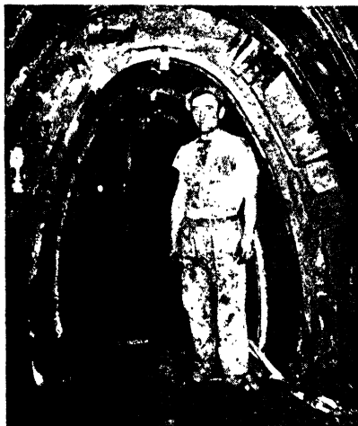
FIG. 55.—Safety lamp (extreme left) kept burning in heading of Chicago sewer tunnel to determine presence of harmful or explosive gas. Lamp goes out when normal oxygen content of air is disturbed.
