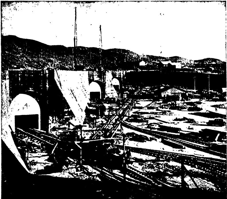
FIG. 115.—Track layout at downstream portals of Fort Peck Dam diversion tunnels, an example of well-laid track. Haulage was by trolley locomotive; 36-in. track gage; 56-lb. rail. (U. S. Engineer Dept. Photograph.)
