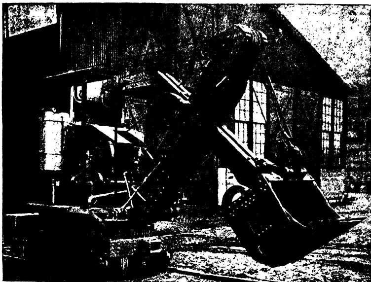
FIG. 76.—An Osgood 1-yd. air-powered full-revolving shovel used in mucking out a 17-ft. tunnel.
