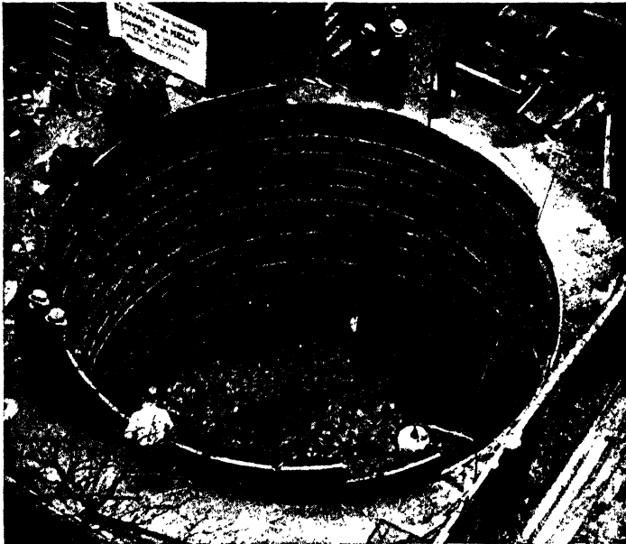
FIG. 65.—A 26-ft. shaft, steel-plate lined, being sunk through blue clay for the Chicago Subway. Excavation was easy with a clamshell bucket handled by a crane. ( Wide World Photograph. )
