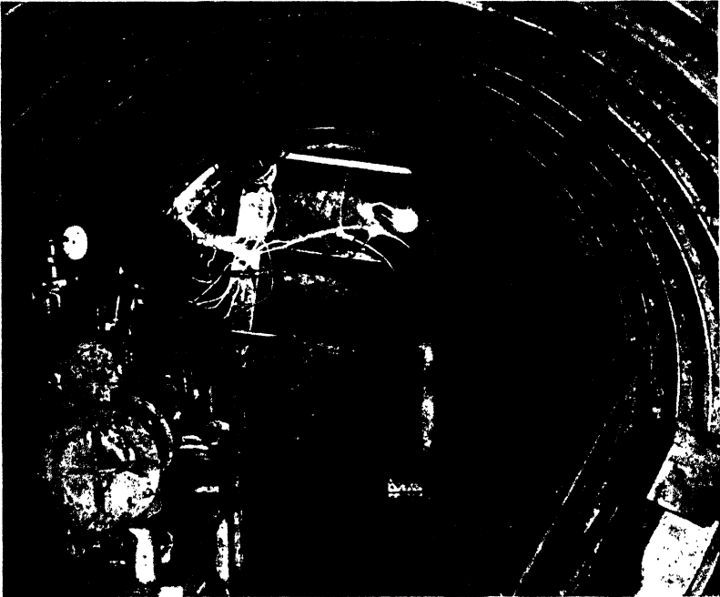
FIG. 237.—Small shield-driven tunnel with primary lining of steel plates and ribs. Hydraulic pressure for operation of the shield is created by air-driven pump in foreground, kept within 50 ft. of the shield. Note how this particular shield has rolled to the right. (Courtesy of Commercial Shearing & Stamping Co.)
