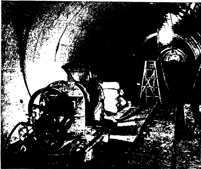
FIG. 362.—Grout machine in operation, Detroit water tunnel.
