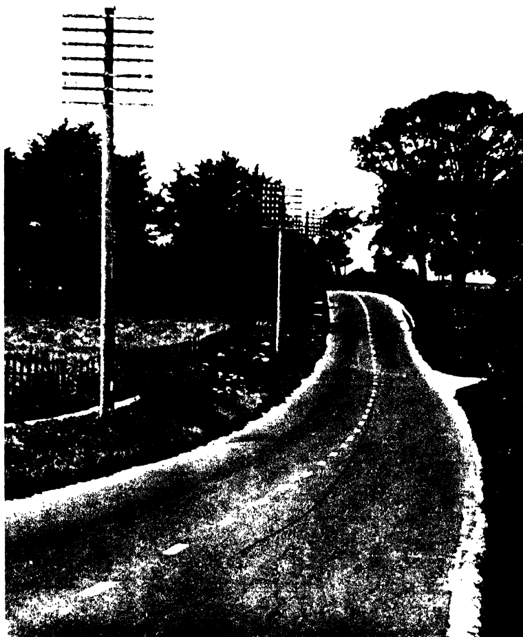
Fig. 19.—Limestone Cold Asphalt Surfacing on A.27, Chichester-Arundel Road, near Crocker Hill. Laid June 1930. Photographed 1945.
