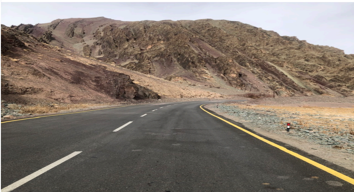
Figure C18: Study of EIA due to fresh laying of AC pavement on a hill road at Leh, Ladakh at an altitude of 16000 ft.
