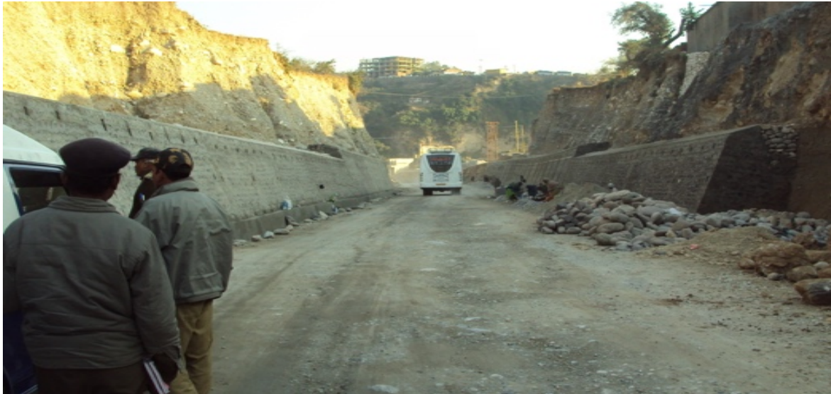
Figure 3.2 Box cut at km 1 near railway tunnel (Source: Author's Field Survey)
