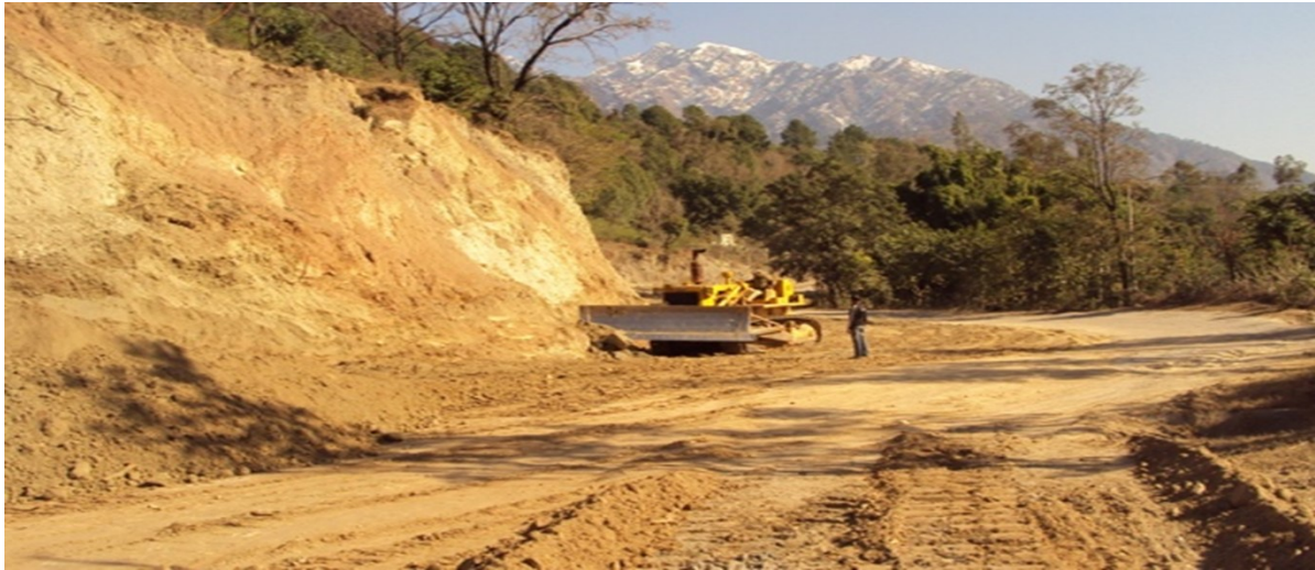
Figure 3.3 Dozer clearing a slope on hill side (Source: Author's Field Survey)
