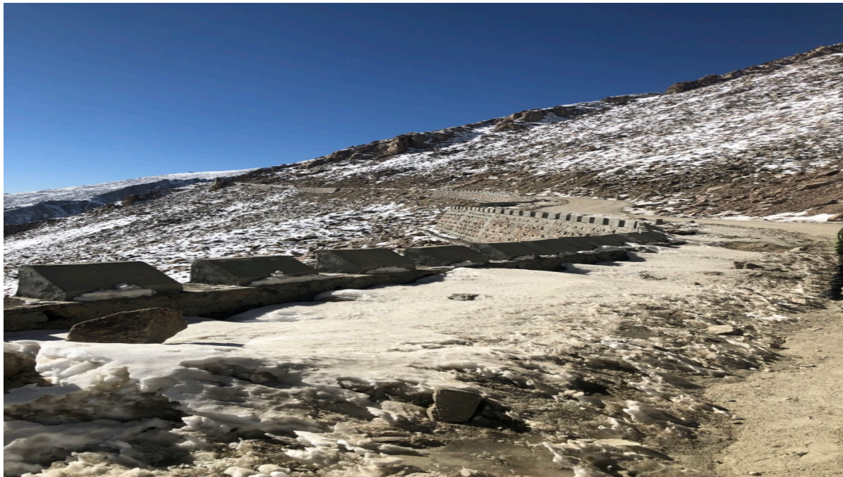
Figure C1: A retaining wall on a snow-clad hill road under construction
