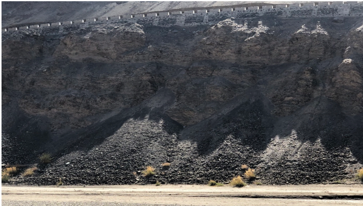
Figure C21: Study of landslide due to rains on a hill road along River Indus in Ladakh.
