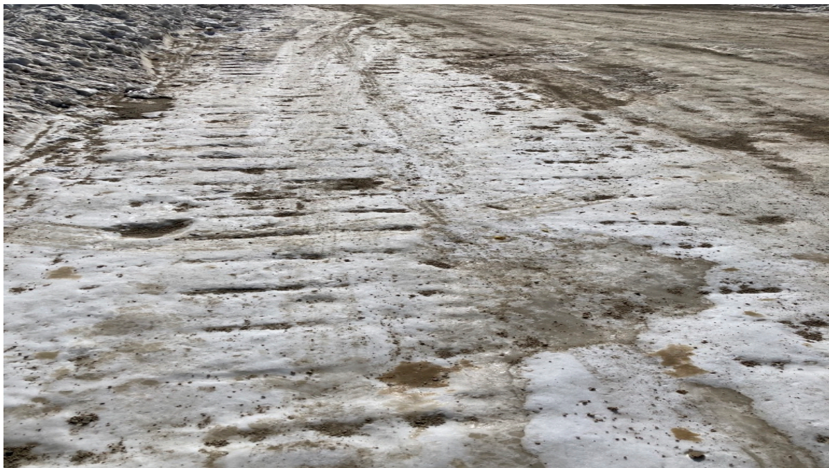
Figure C4: Dozer Marks on the road after snow clearance
