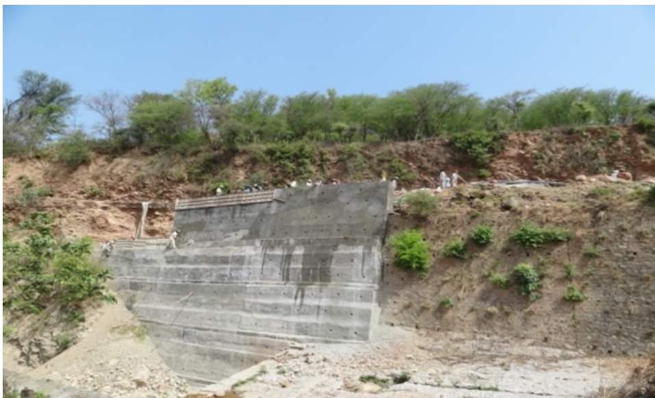
Figure 3.16 The Retaining Wall Being Constructed at km 18 (Source: Author's Field Survey)
