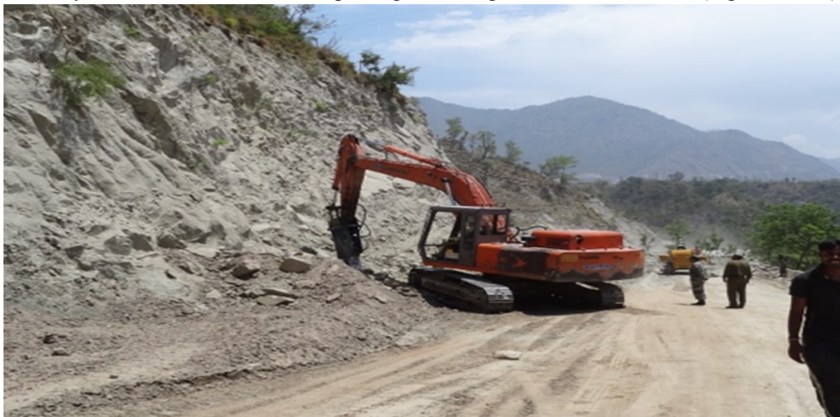
Figure 3.6 A Rock Breaker Operating on Last Stretch (Source: Author's Field Survey)
