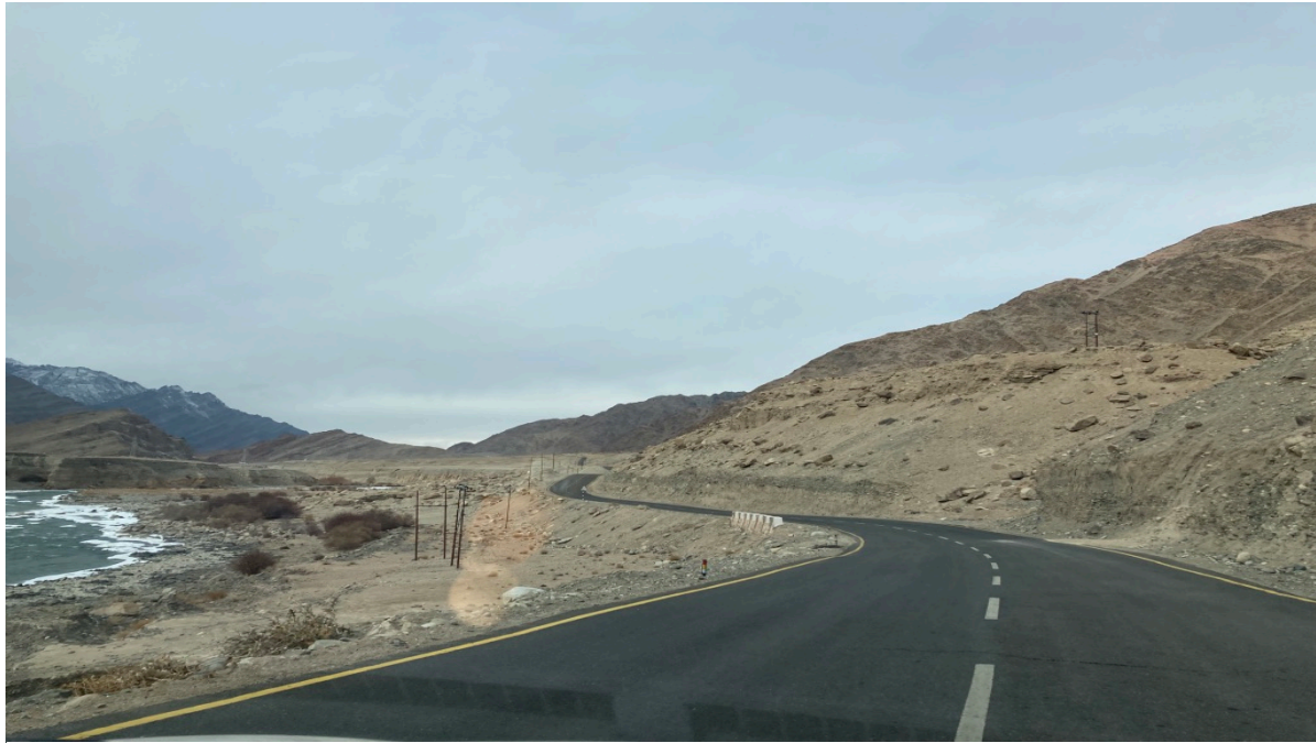
Figure C19: Study of EIA including impact on river due to a hill road construction at Leh, Ladakh at an altitude of 16000 ft.
