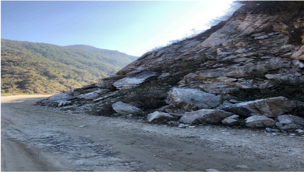
Figure C17: Landslide triggered by rains on a hill road in Uttarakhand
