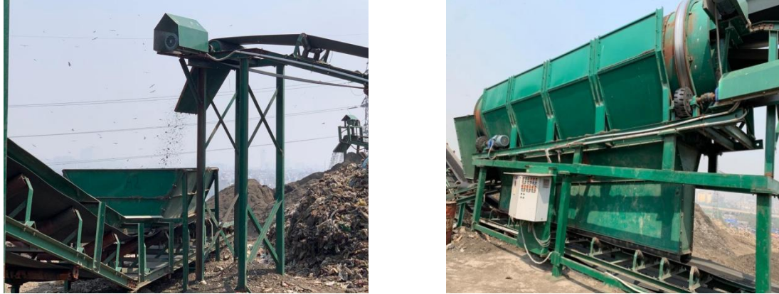
Fig. 2.10 Waste processing through trommel screens at landfill site
