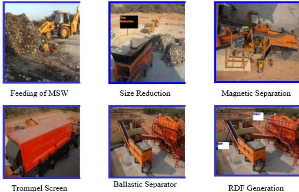
Fig. 2.9 Preparation of RDF at Jaipur RDF plant of UTCL
