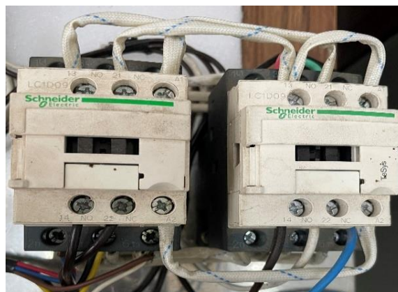
Figure 3.19 Contactor switch
