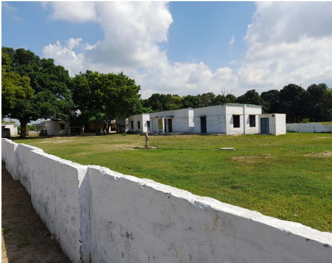
Picture 10: Secondary school with difficulty of accessibility - Bahraich
