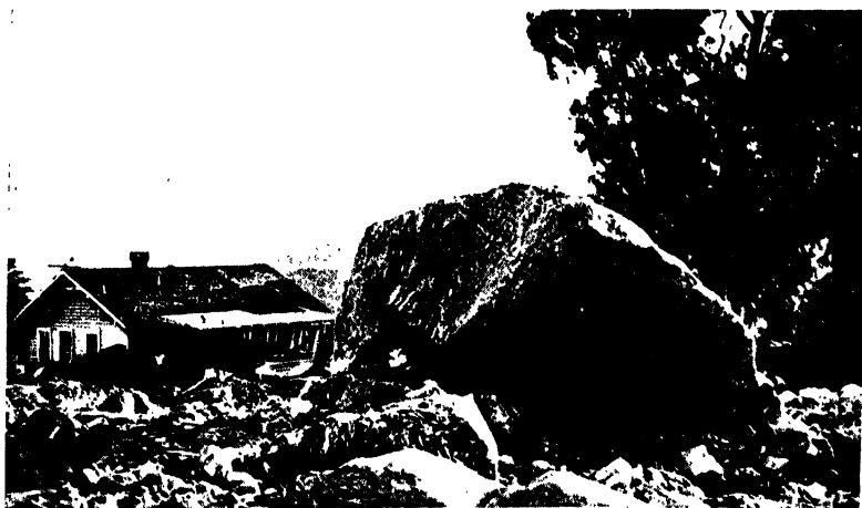
FIG. 21.—Destruction of highway-maintenance station, near La Crescenta, California, caused by flood from burned-over mountain area, Dec. 31, 1933.
