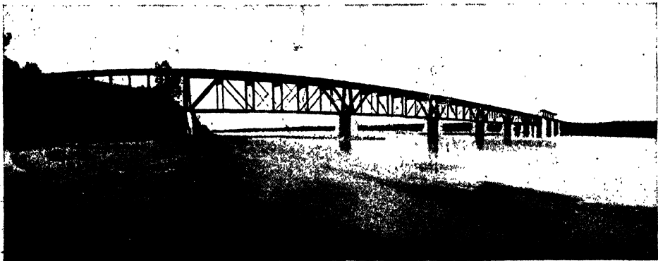
NORTH BATTLEFORD BRIDGE, ONE OF THE LONGEST IN CANADA
