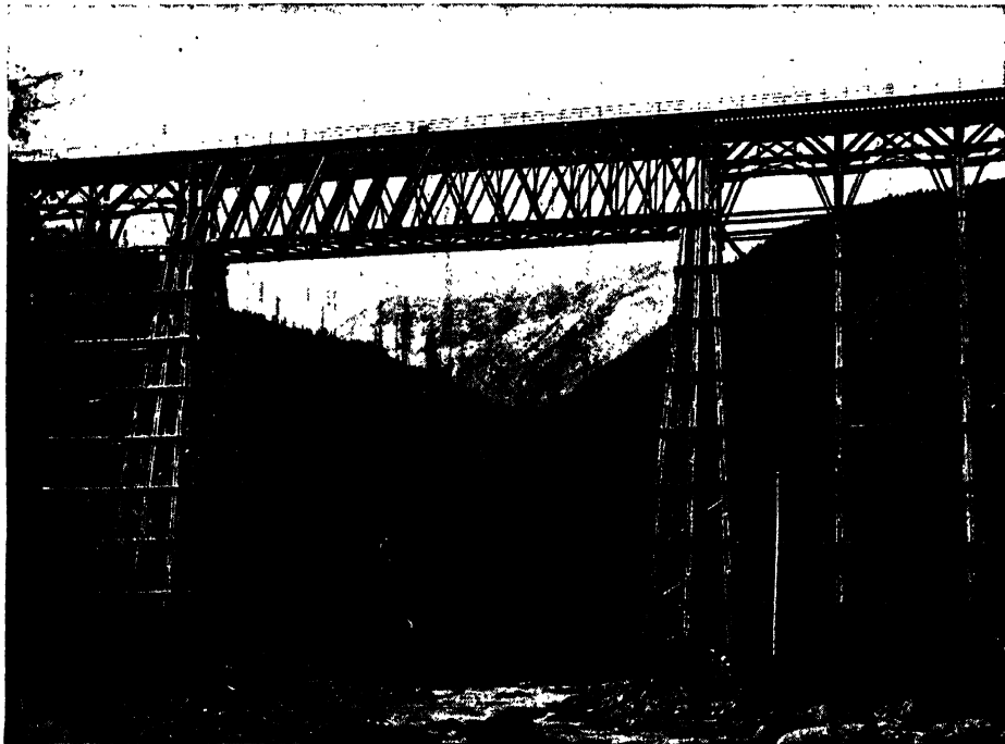
MOUNTAIN CREEK BRIDGE, CONTAINING ONE AND A HALF MILLION FEET OF TIMBER
