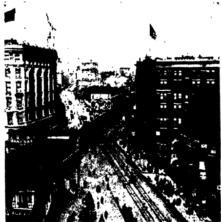
ELEVATED RAILWAY CROSSING BROADWAY
