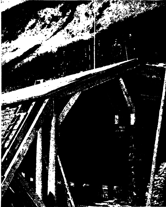
SNOW-SHED ON THE CANADIAN PACIFIC RAILWAY
