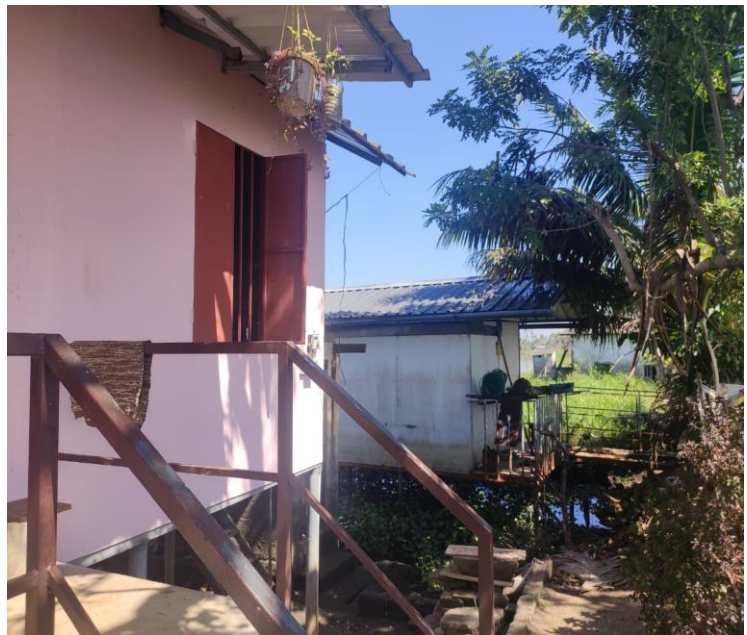
Figure 3. 15: Temporary shelter built on large pillars
