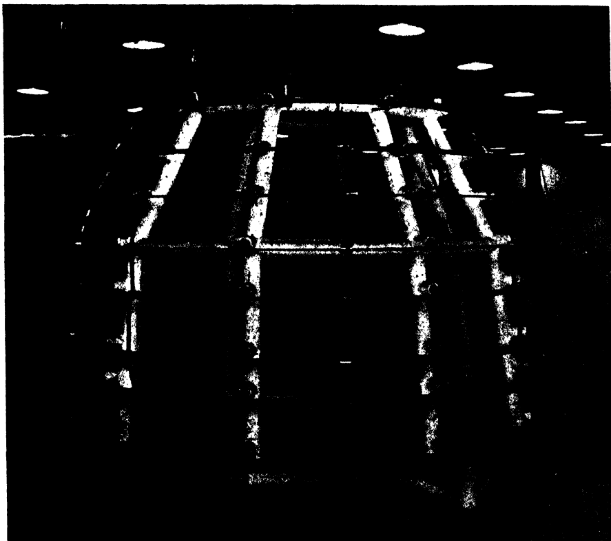
FIG. 94. Mock-up Skeleton with Contour Templates.
