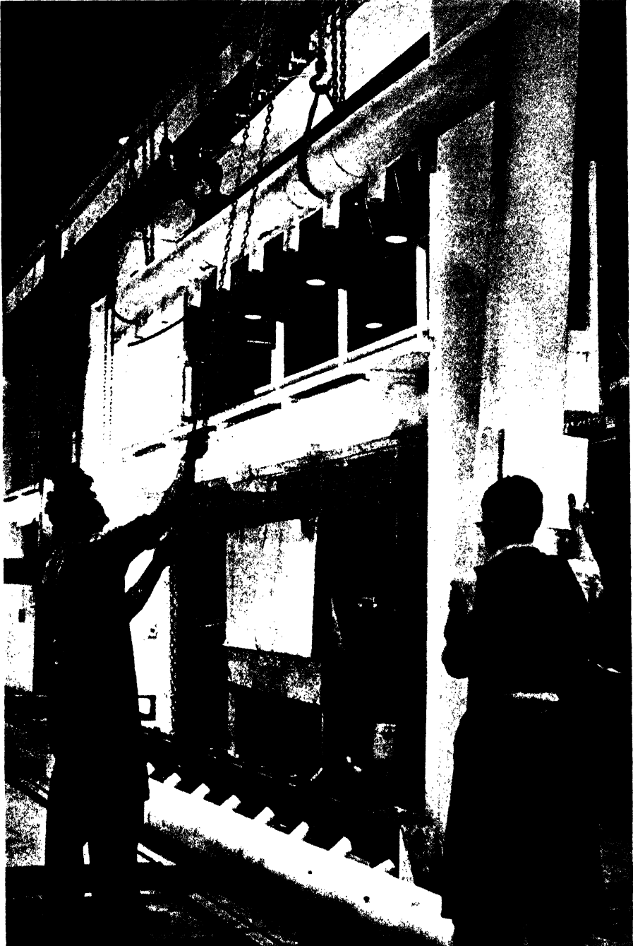
FIG. 81. Moving a Jig Frame into the Master Tooling Dock.
