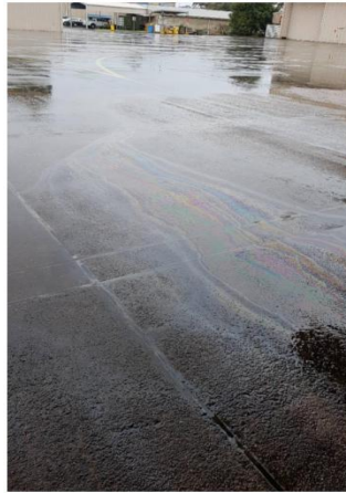
(a) Leaked oil from aircraft with rainfall runoff
