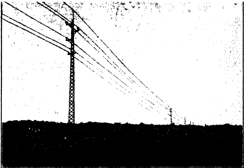
FIG. 48.—Typical transmission line carried on latticed steel masts.
