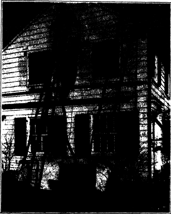
Fig. 14. Pneumatic Method of Insulating Existing Walls with Mineral Wool Courtesy of Johns-Manville, New York, N. Y.
