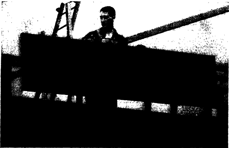
Fig. 22. Application of 2x8 Structural Insulating Board Sheathing Courtesy of United States Gypsum Co., Chicago, Ill.
