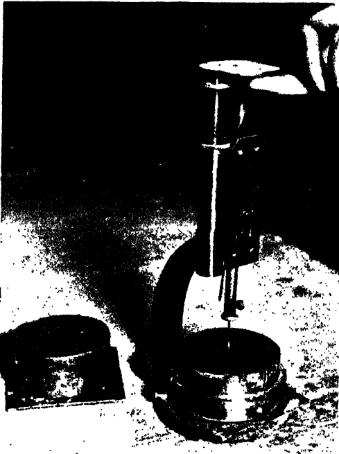
Fig. 42.—VICAT APPARATUS FOR SETTING TIME
