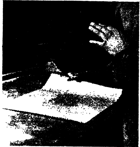
Fig. 35.—SIEVE TEST FOR CEMENT
