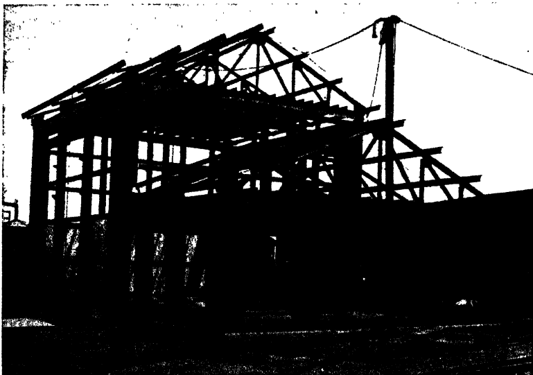
FIG. 138.—Steel structure of pipestill. (A. J. Smith Engineering Company.)
