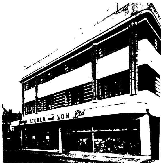
A SUBURBAN STORE—SIDE AND REAR
