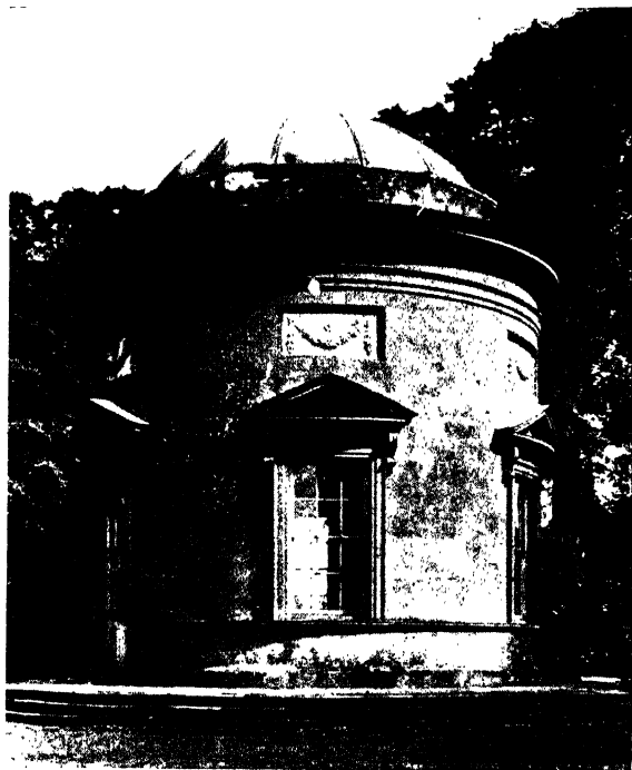
82 Croome Court, Worcestershire: the Garden Room, circa 1766
