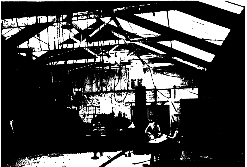
(Below) Interior of the studio of Cricks and Martin at Waddon New Road, Croydon
