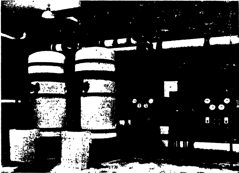
Fig. 19. —Two ELECTRODE WATER HEATERS OPERATING AT HIGH VOLTAGE
