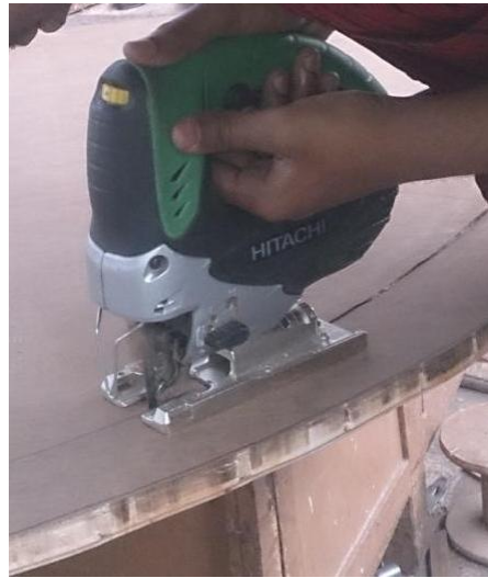
Fig. 5.2 The fabrication of parabolic trough plywood base using jig saw
