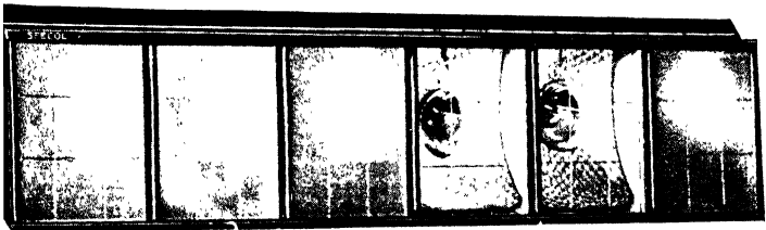
SECTION OF A FLOAT, OR FOOTLIGHTS, SHOWING LAMPS WITH REFLECTORS AND GELATINE COLOUR MEDIUMS
