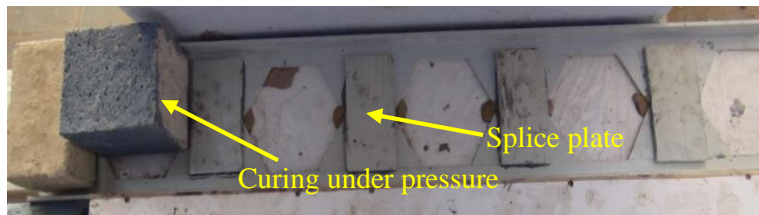
(c) Installation of splice plate over T-sections
