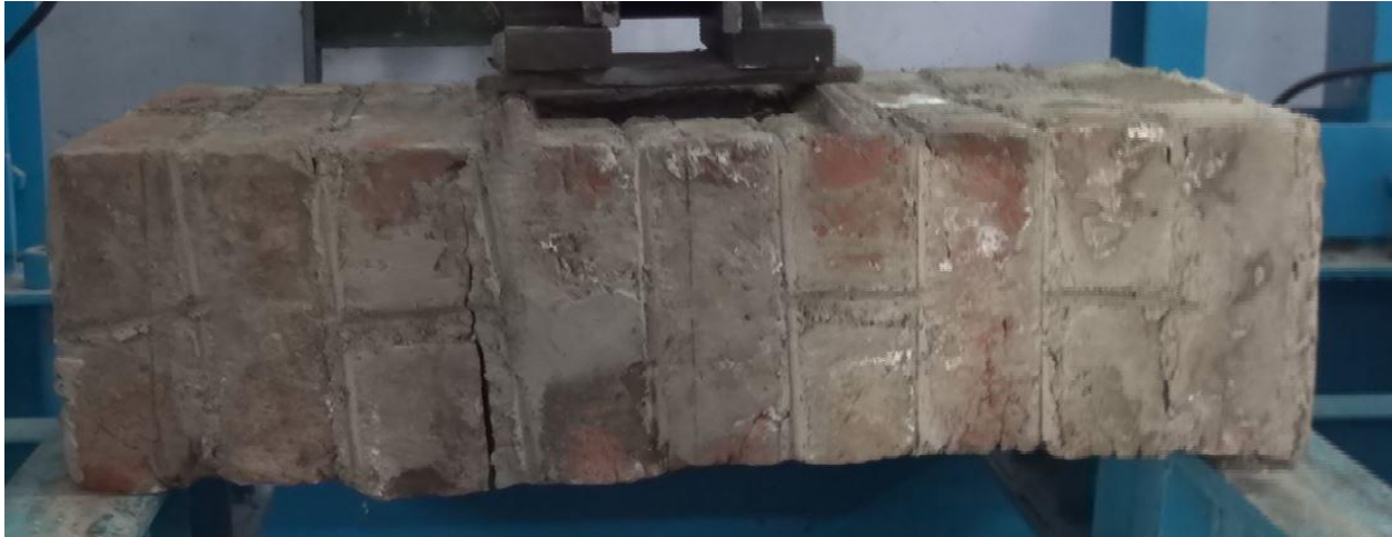
Fig. 5.13 Failure pattern of control masonry wall with opening (Series #2 specimen)
