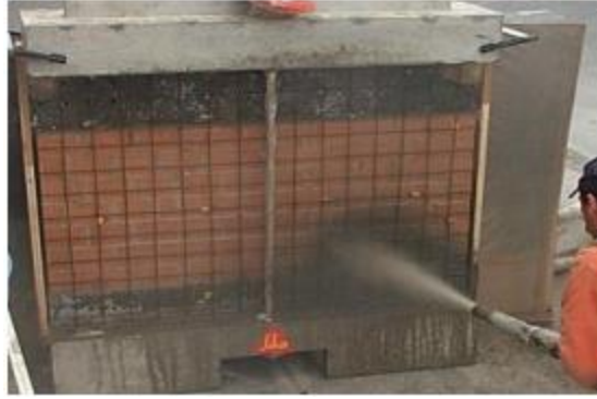
Fig. 1.1 Applying Shotcrete [10]
