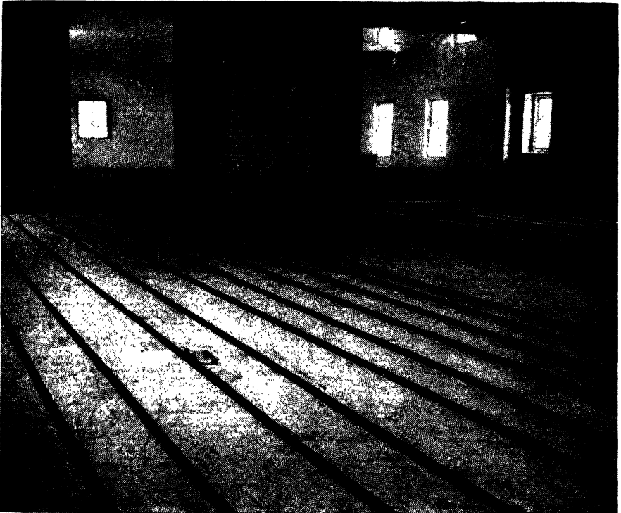
FIG. 2-19.—Radiantly heated garage and shop. ( Bethlehem Steel Co. )
