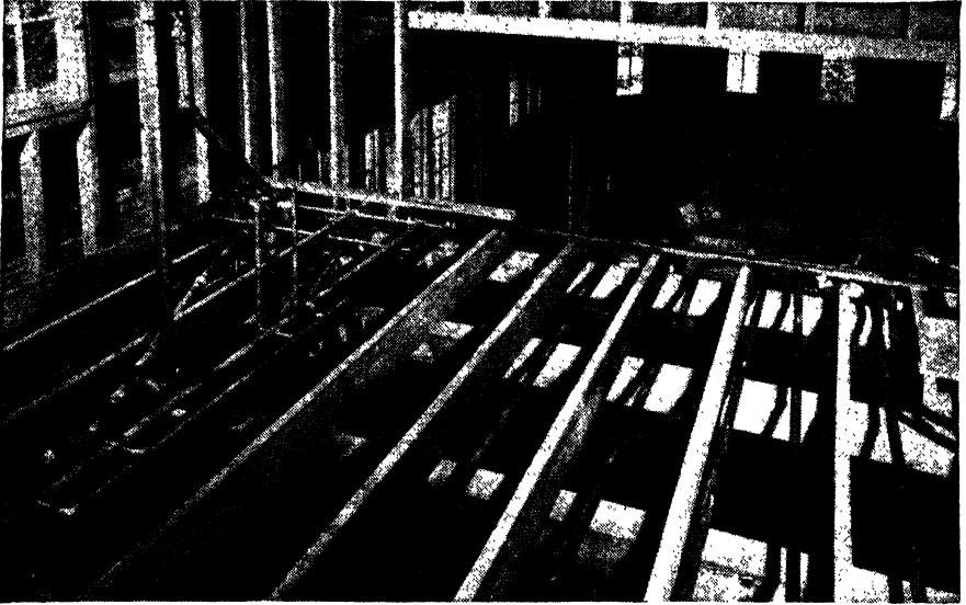
FIG. 4-10.—Residential second-story floor construction. ( Bethlehem Steel Company. )
