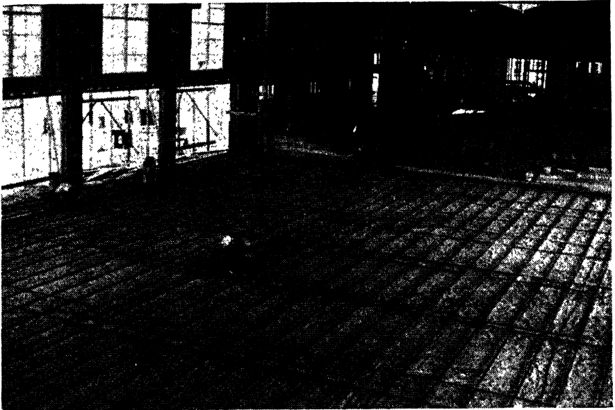
FIG. 3-25.—Floor installation in chapel. ( A. M. Byers Company. )
