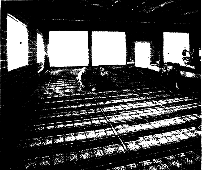
FIG. 2-20.—Installing steel pipe coils for radiantly heating a firehouse. ( Bethlehem Steel Co. )
