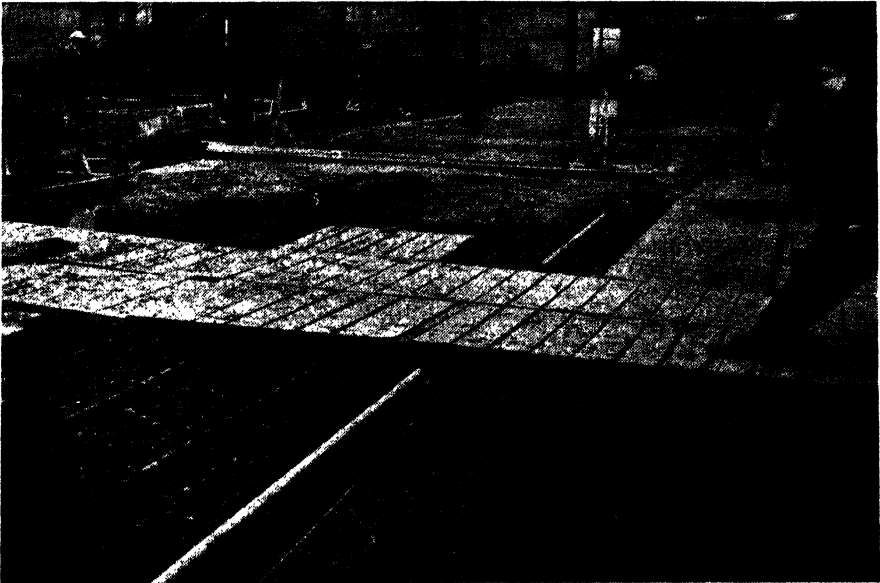
FIG. 8-8.—Pouring floor slab in sections. ( A. O. Smith Corporation. )
