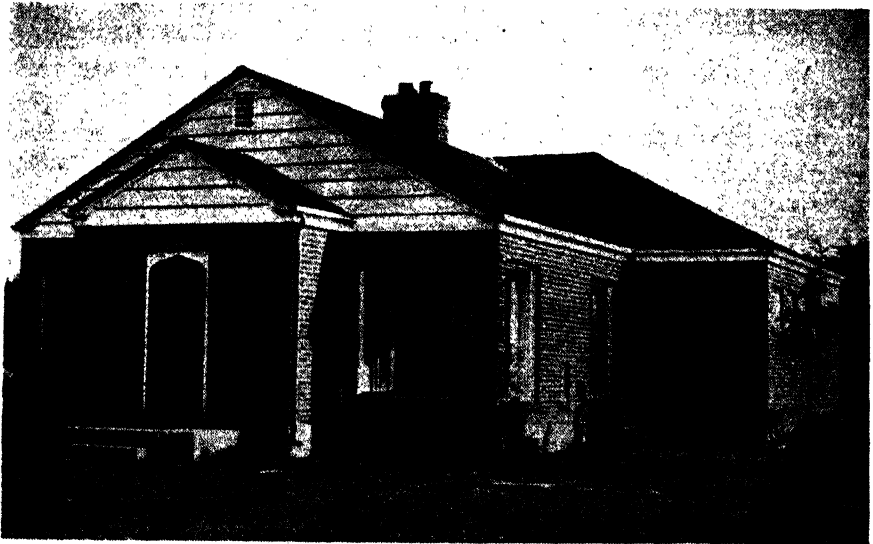
FIG. 9-6.—Radiantly heated and summer air-conditioned bungalow. ( Bethlehem Steel Company. )
