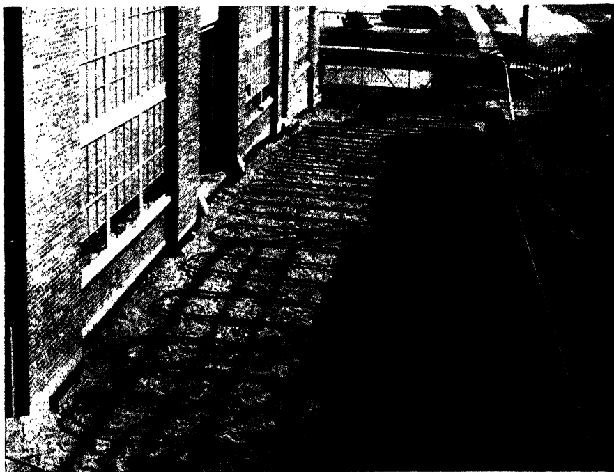
FIG. 8-38.—Snow-melting application in driveway. ( National Supply Company. )
