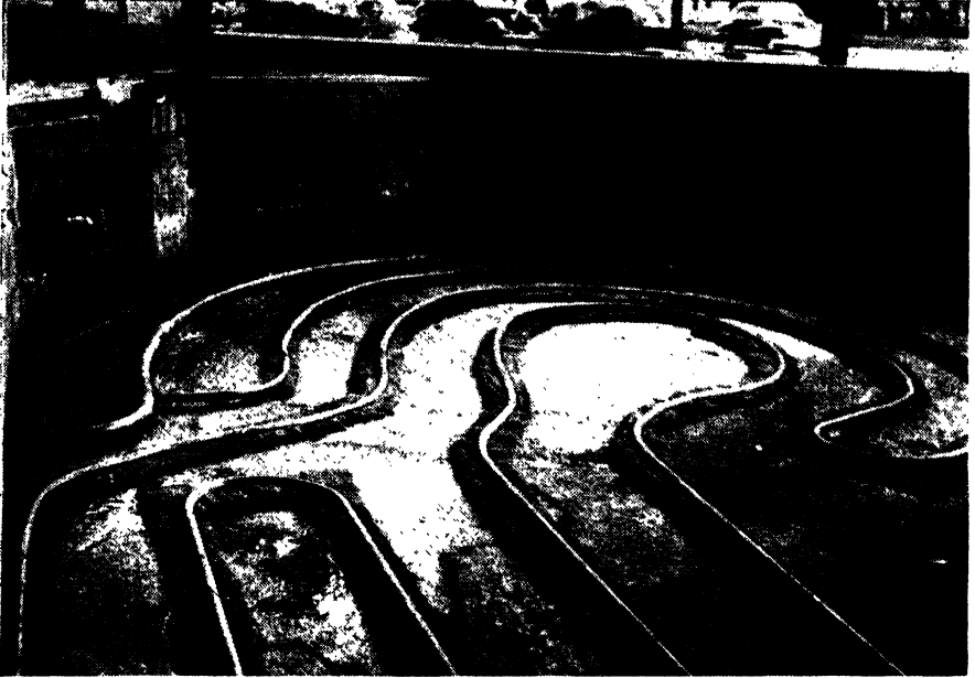
FIG. 3-23.—Floor coils in service station. ( Chase Brass & Copper Co., Inc. )
