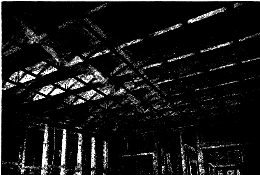
FIG. 4-18.—Wrought-iron ceiling installation. ( A. M. Byers Company. )
