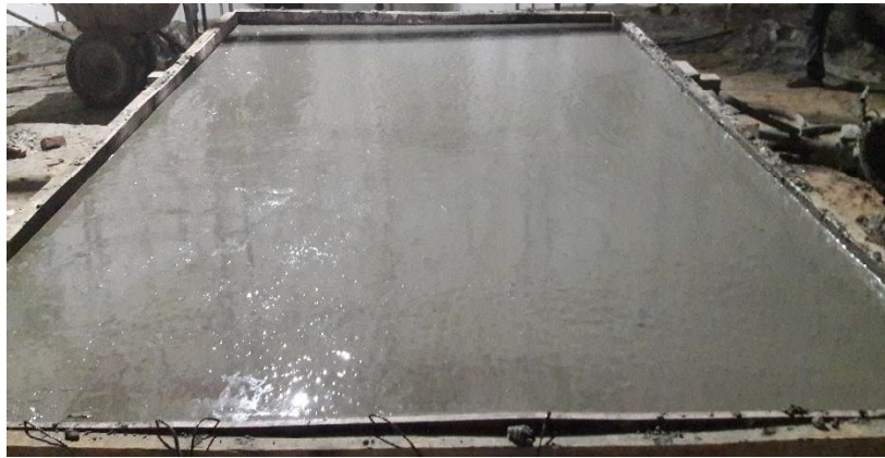
Figure 3.21. Casted bridge deck slab
