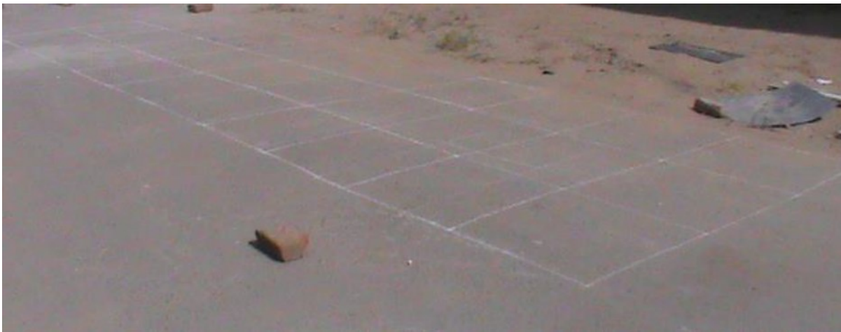
Figure 3.3. Initial demarcation of blocks on existing asphalt pavement before laying of bonding/anomaly conditions
