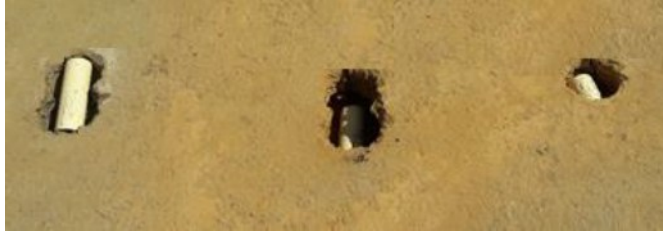
Figure 3.6. PVC pipes placed at the cored locations
