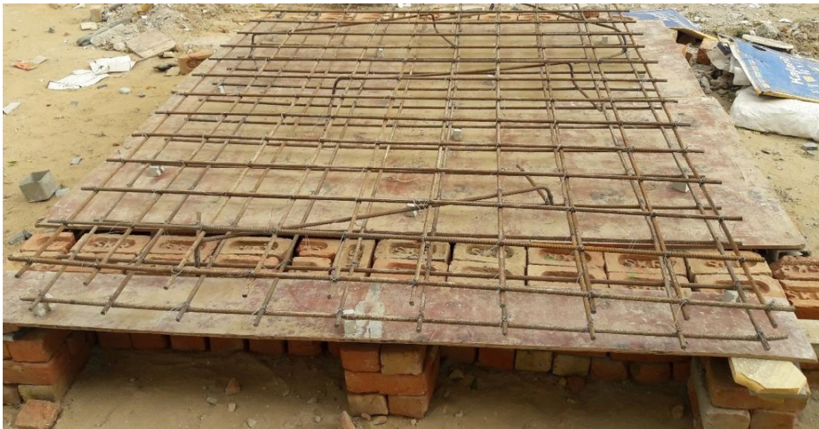
Figure 3.16. Reinforcement mats laid for the construction of concrete bridge deck slab
