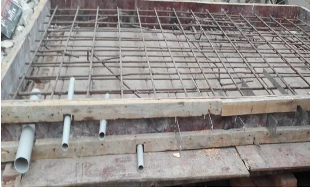
(a) PVC pipes and steel strips
