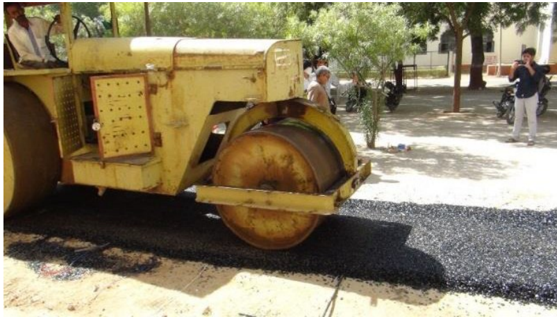
Figure 3.10. Compaction of constructed test section using smooth wheel roller
