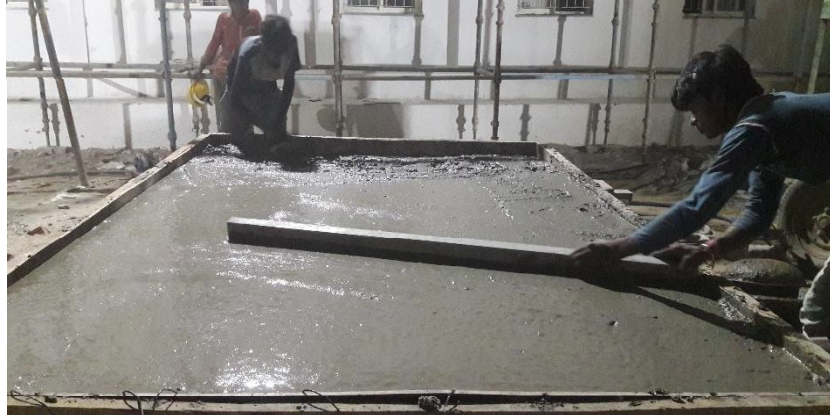
Figure 3.20. Final finishing while casting slab
