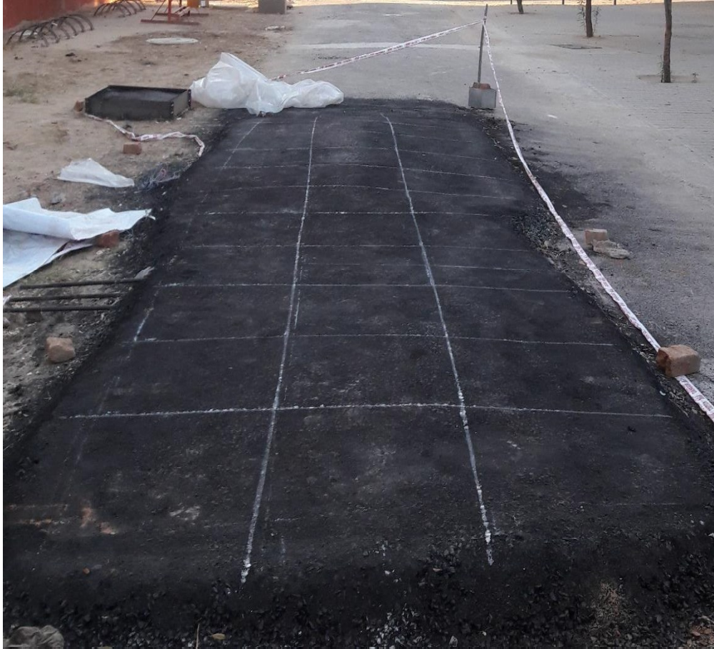
Figure 3.13. Constructed in-situ asphalt pavement test section
