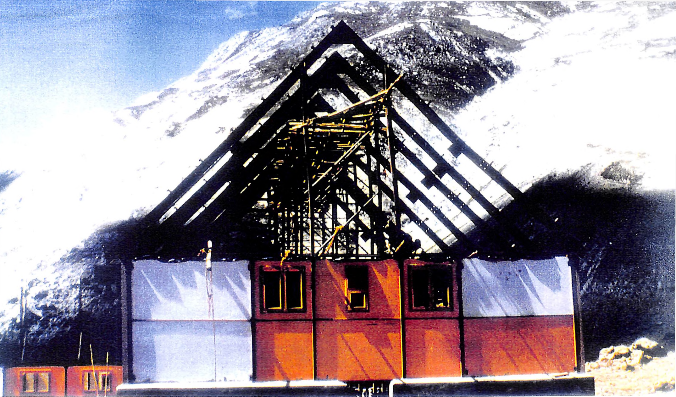
PLATE 5.13 ASSEMBLY OF STRUCTURE
