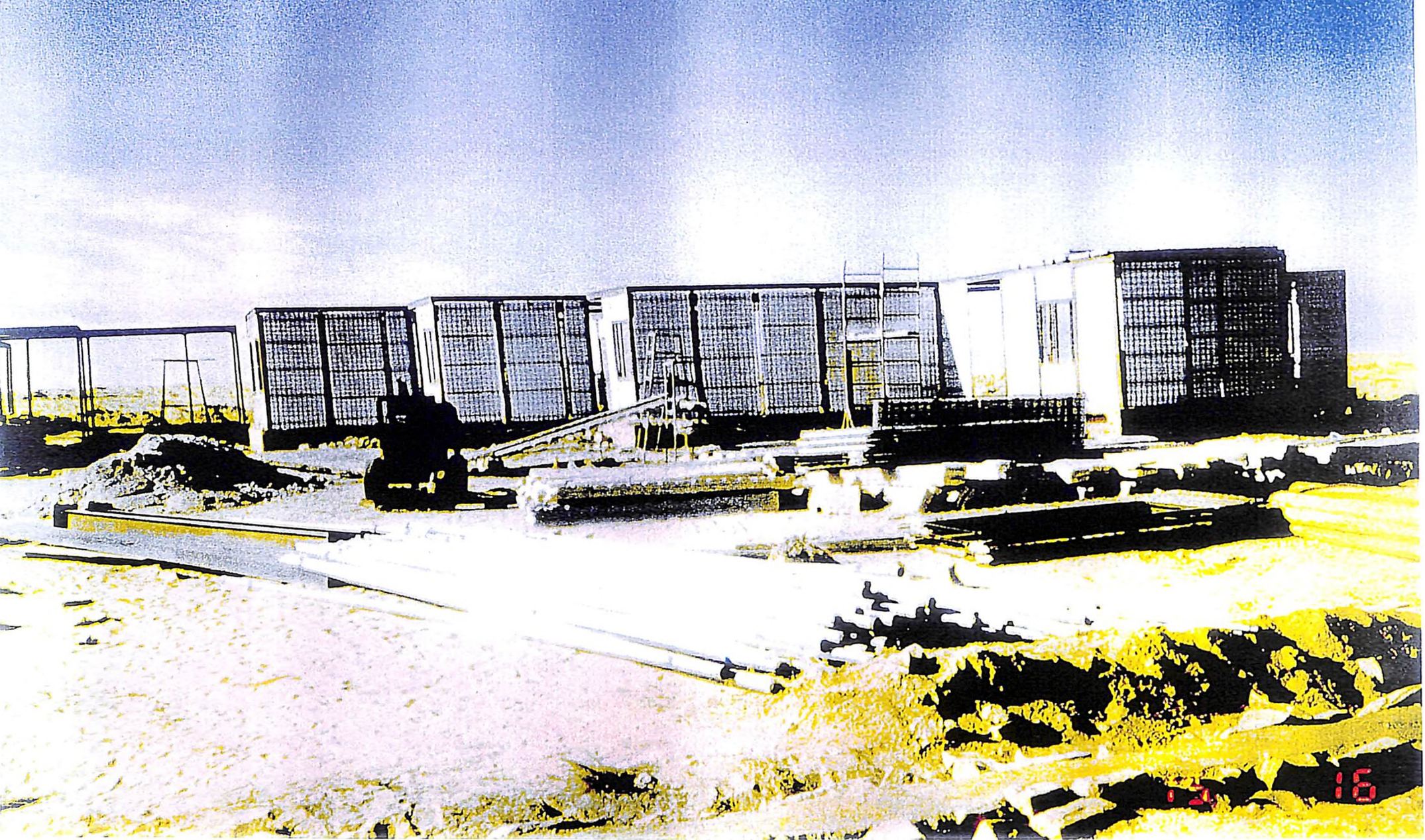
PLATE 4.5 SANDWICH PANEL ASSEMBLY AND ERECTION
