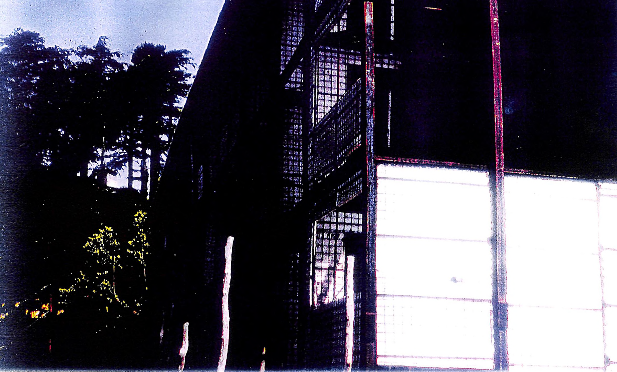
PLATE 6.5 POSITIONING OF SANDWICH PANEL
