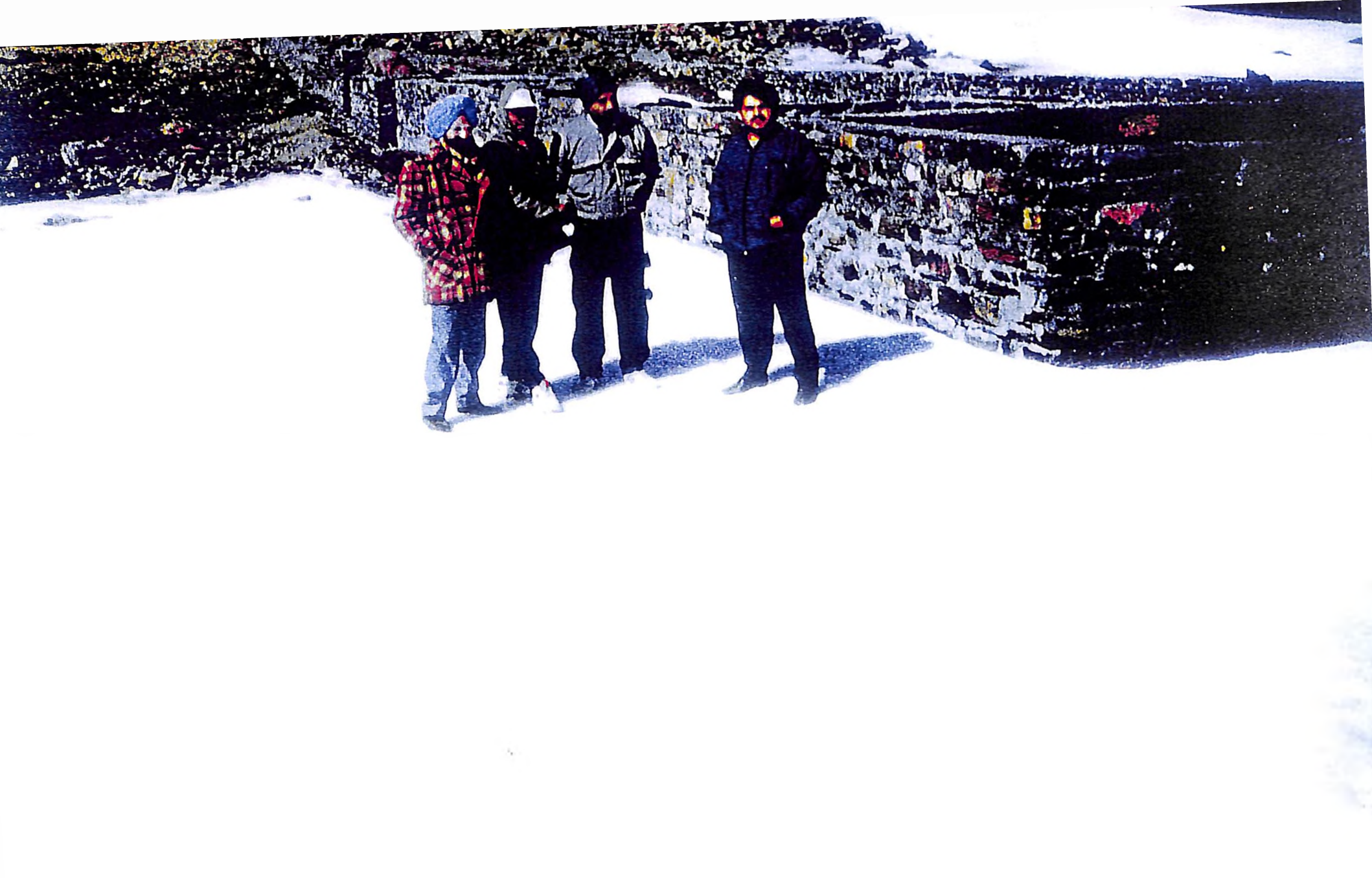
PLATE 5.9 PLINTH OF PROPOSED BUILDING (VIEW DURING SNOW)
