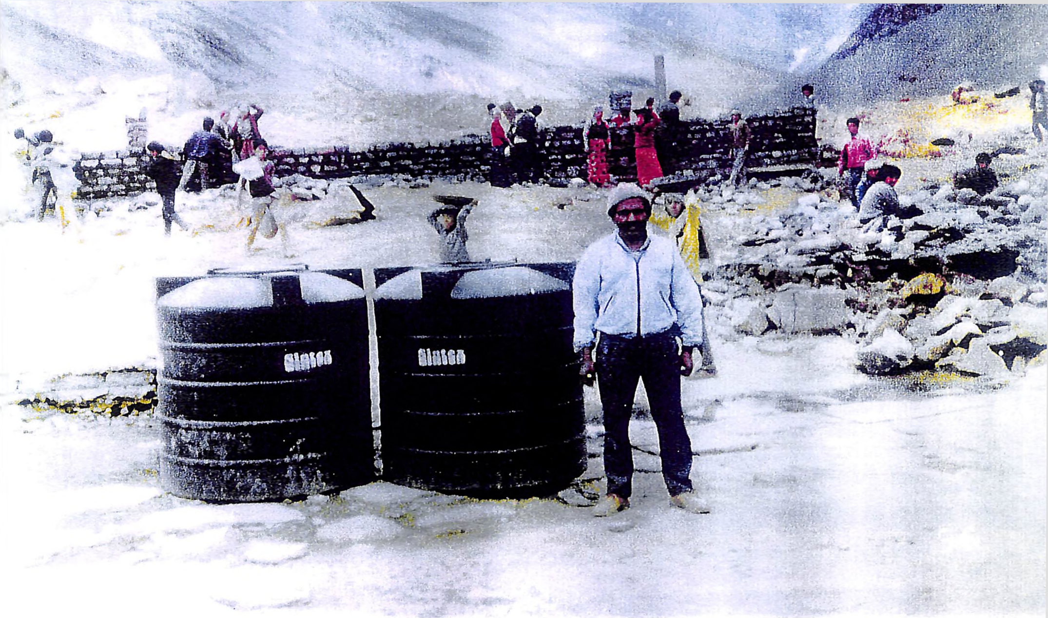
PLATE 5.12 PLINTH OF PROPOSED BUILDING (UNDER CONSTRUCTION)
