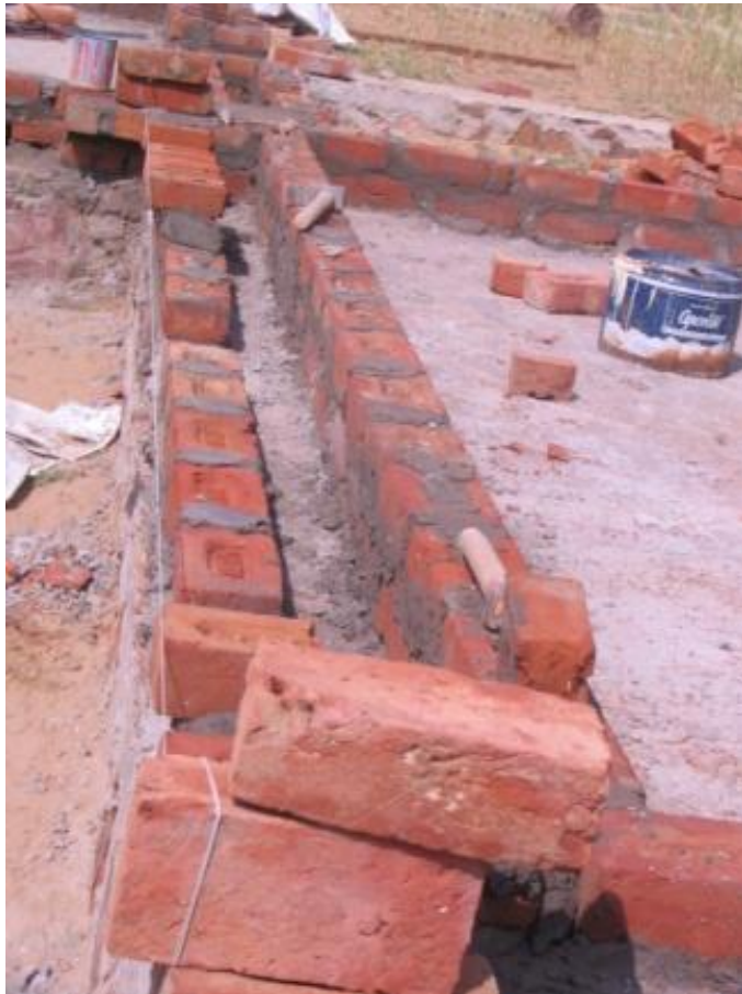
Fig. 4.12 View of courses of brick cavity wall with brick projections (a) View of first course (b) View of second course
