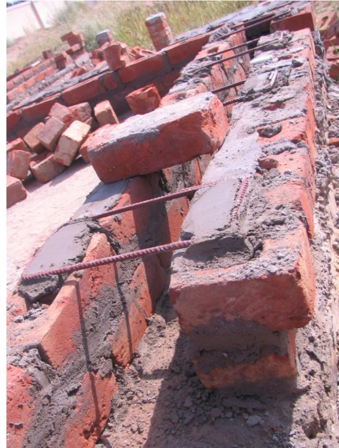
Fig. 4.13 View of brick cavity wall with brick projections under construction (a) View of west wall and south wall (b) View of rectangular mild steel wall ties
