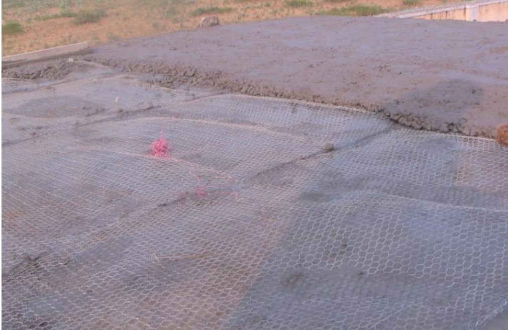
Fig. 4.18 View of chicken wire mesh and concrete layer in hollow roof
