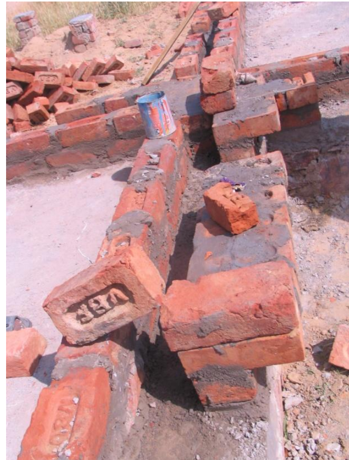
Fig. 4.12 View of courses of brick cavity wall with brick projections (a) View of first course (b) View of second course
