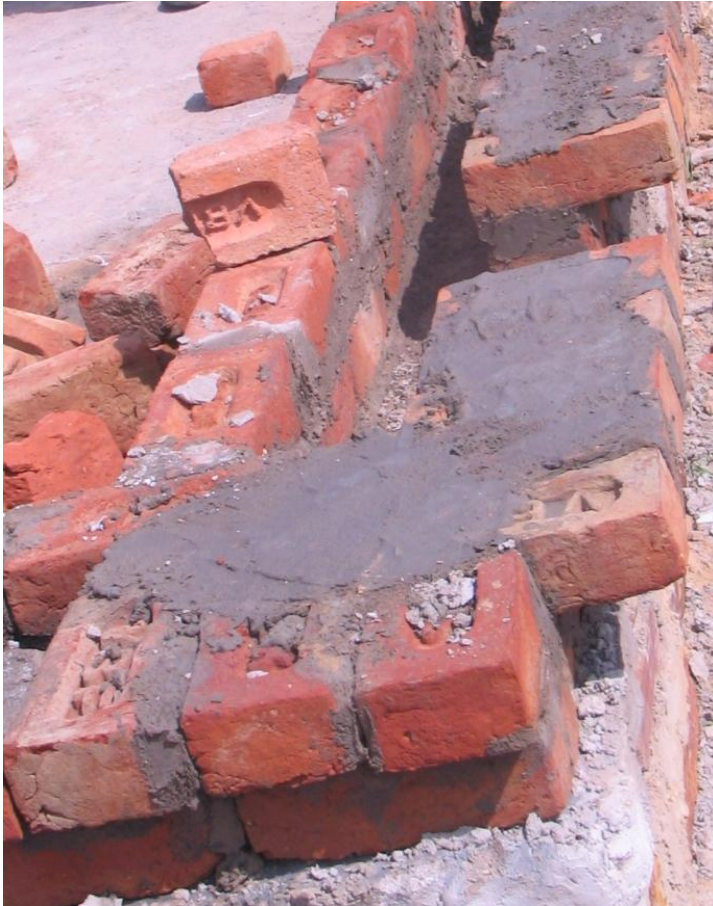
Fig. 4.13 View of brick cavity wall with brick projections under construction (a) View of west wall and south wall (b) View of rectangular mild steel wall ties
