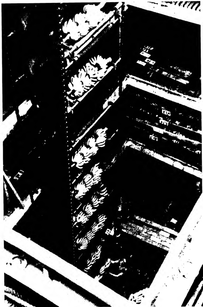
CAREFULLY LOWERED INTO THE HOLD
