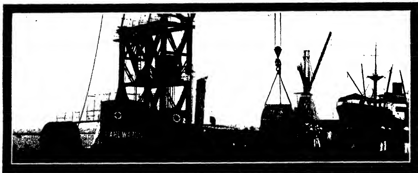
Unloading two drums of Electric Cable at Karachi, each weighing 19 tons 3 cwt., diameter 9 ft. 8 in., width 6 ft. 2 in., the largest and heaviest drums of cable ever imported into India. Sent out by W. T. Henley's Telegraph Works Co. Ltd. for laying across the River Indus. Each contains 4,500 ft., 04 sq. in. 3-core extra high tensile 6,600 volt double wire armoured Underwater Cable.
