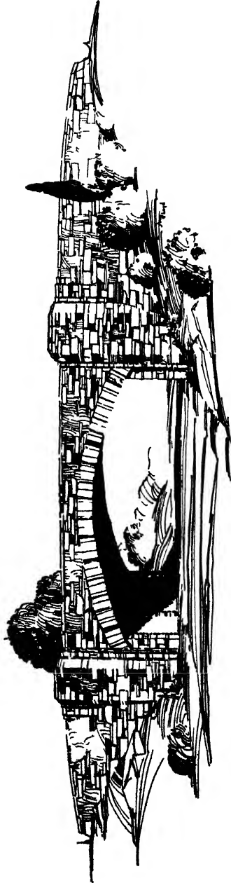
Wellington Underpass —Mt. Vernon Memorial Highway, Washington, D. C. (Rigid frame construction) Gilmore D. Clarke, & Clinton F. Loyd, Architects. J. V. McNary, Designing Engineer, U. S. Bureau of Public Roads
