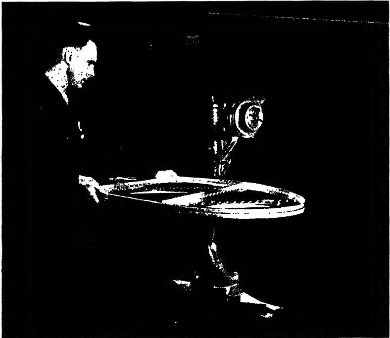
Fig. 7. Air-operated Automatic Punching and Riveting Machine
