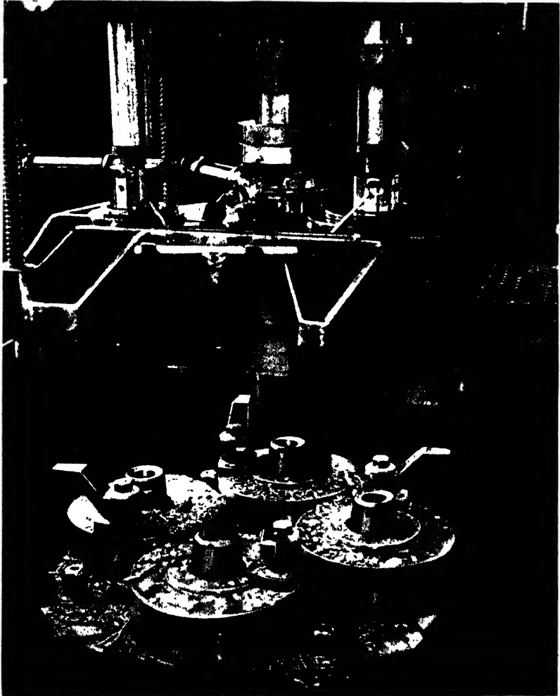
Fig. 14. Boring, Facing, and Turning the Nose Ends of Shells in a Three-spindle Drilling Machine Equipped with an Indexing Table
