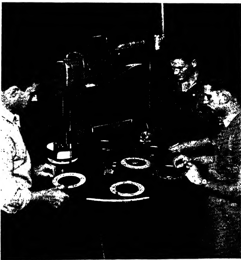
Fig. 10. Multiple Riveting Operation that Employs an Indexing Work-carrying Dial
