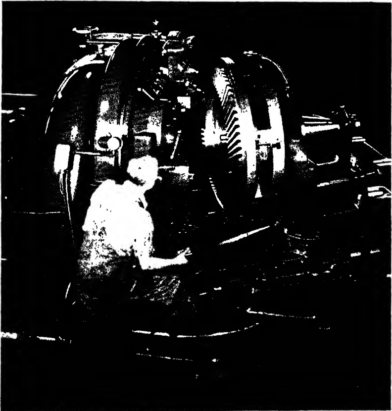
Fig. 10. Cutting the Teeth of a Spiral Bevel Gear
