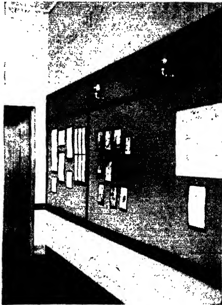
FIG. 117.—The two photocells mounted on the rear wall of this school-room control the illumination within the room in accordance with the degree of natural light available.
