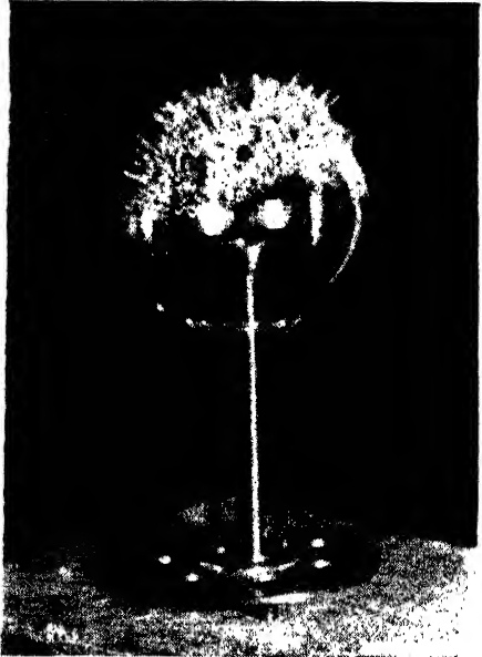
FIG. 281. Glass rubbed with tin-amalgam chamois.
