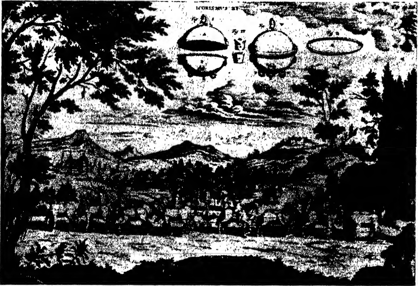
FIG. 98. The Magdeburg hemispheres experiment.
