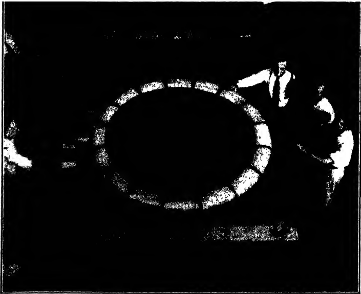
FIG. 160. 100-MEV BETATRON WITH THE TOP POLE REMOVED, SHOWING VACUUM TUBE.
