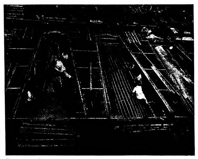
Fig. 287. Aluminum framework and skin being assembled on a Consolidated B-24
