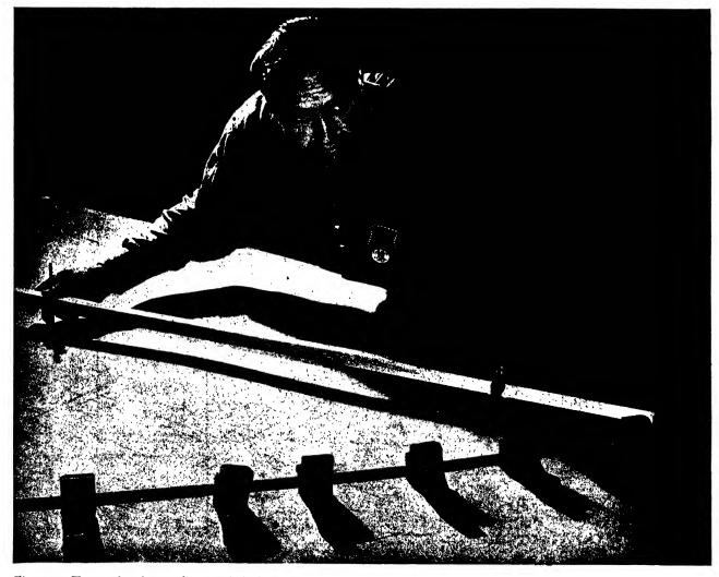
Fig. 380. Trammel points, spline, and ducks in use
