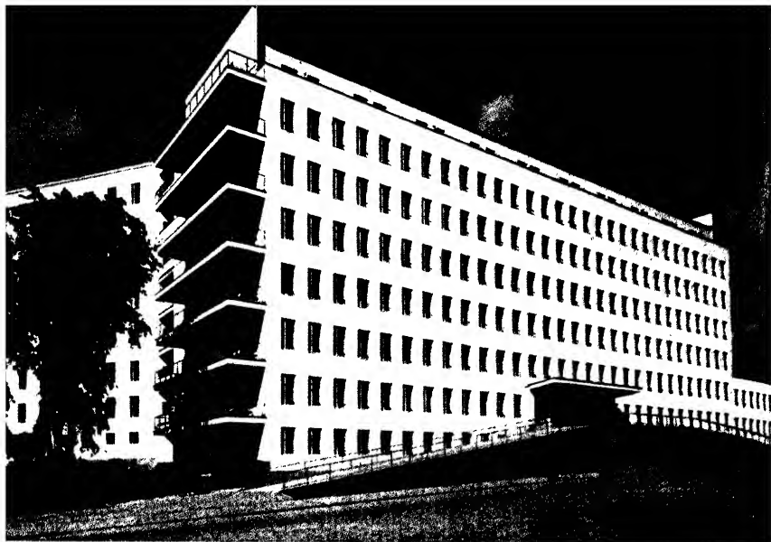
48.—A hospital built at Turku, Finland, before the war. The balconies are deep enough to take beds, the sills of the windows are kept low. The building depends for its effect upon the proportions of the openings and upon the pattern of openings in the wall they create. There is nothing adventitious or unnecessary in the design, yet it is gay and elegant.
