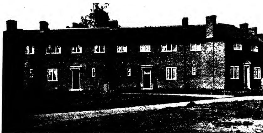
3.—Typical of the housing erected between 1919–39. The Ministry of Health were able to impose minimum standards in construction and floor area by means of the subsidy. The standard—in design, amenity, and lay-out—varied with the wealth and interest of each housing authority.
