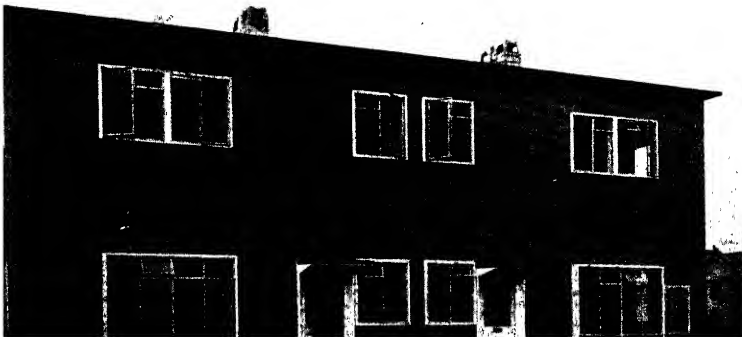
7.—The factory-made house. This pair of houses erected at Edinburgh in 1945 was built from large units which were assembled on the site. Good houses can be built by prefabricated methods.
