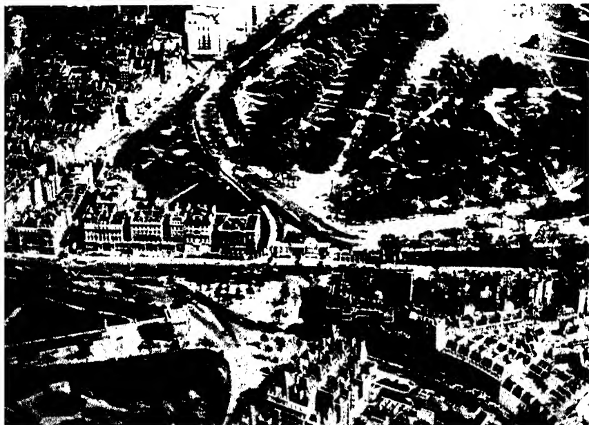
49.—St. George's Hospital, Hyde Park Corner. This hospital is surrounded on three sides by roads which carry heavy traffic and suffers through vibration and noise. Its site does not easily permit expansion.
