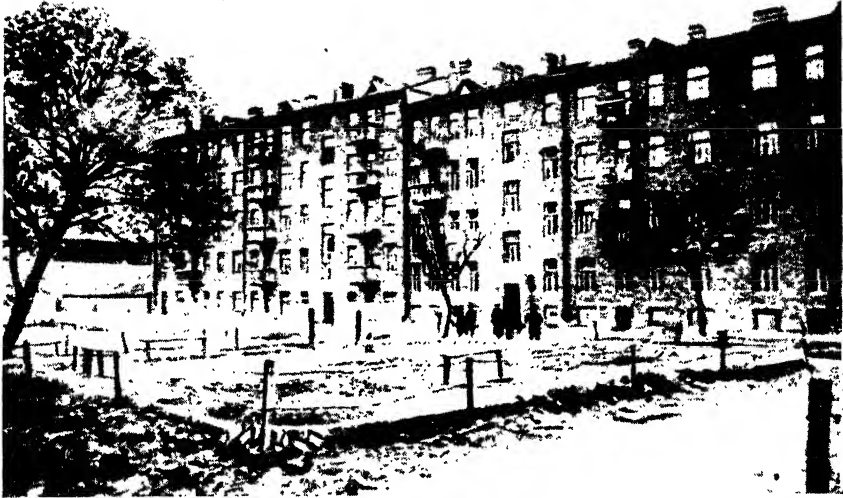
House No. 92/1 on the corner of Sampsonievsky Prospect and Serdobolskaya Street in Petrograd where in Flat No. 42 Lenin lived in hiding after his return from Finland up to October 25 (November 7) 1917
