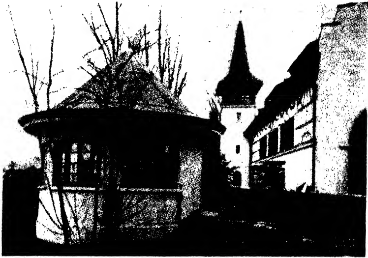
Fig. 75.--The exterior of the pumping works shown in Fig. 74
