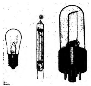
Fig. 15.9.—Filamentary reference elements.
