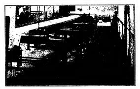
Stentering Machine driven through Crofts Improved Variable Speed Gear
