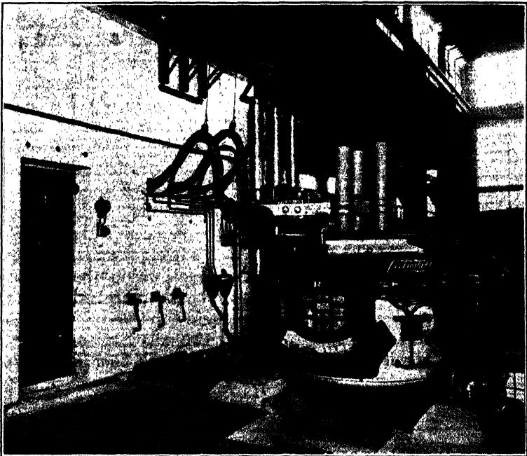
FIG. 38.—Electric Steel-melting Furnace.
