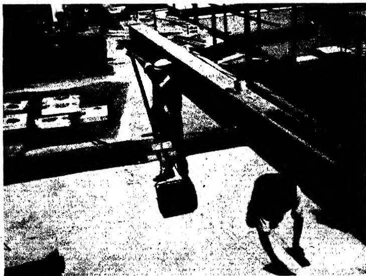
FIG. 78. APPLICATION OF WHITE SPAR CHIPPINGS OVER AN ASPHALTE ROOF SURFACE TO PROVIDE A HEAT-REFLECTING SURFACE
