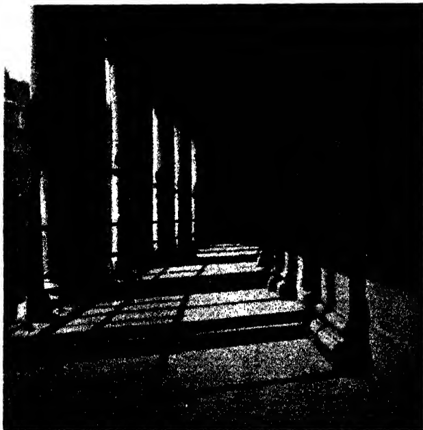
FIG. 89. ILLUSTRATING THE LONGEVITY OF NATURAL ASPHALTE MASTIC Photograph taken at the Gaiety Theatre, London, in 1939, nearly fifty years after the surface was laid.
