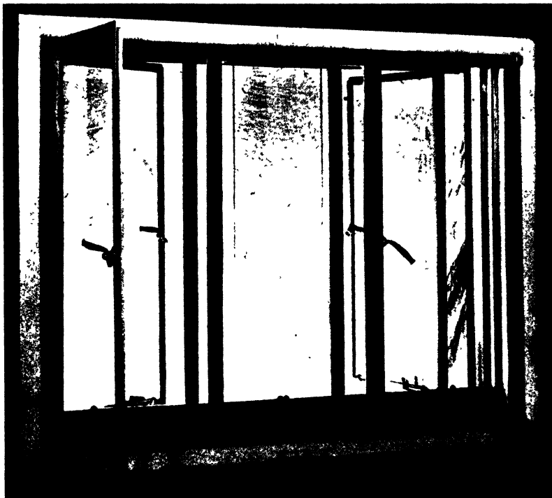
FIG. 105. A MORE ELABORATE DESIGN OF SOUND-INSULATING WINDOW
